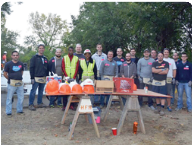
Construction volunteers and Kirby Family at the site of their home at 7209 East 45th Street in Lawrence
