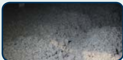
Insulation was put into the basement.
