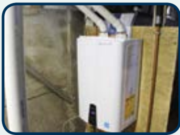
A new water heater was installed.
