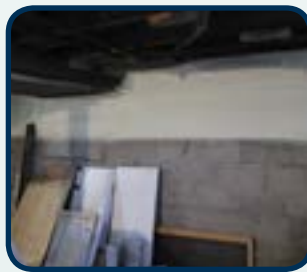
Foam insulation was put throughout the basement.
