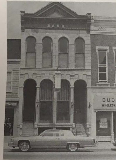
WEST MAIN STREET (South Side)
