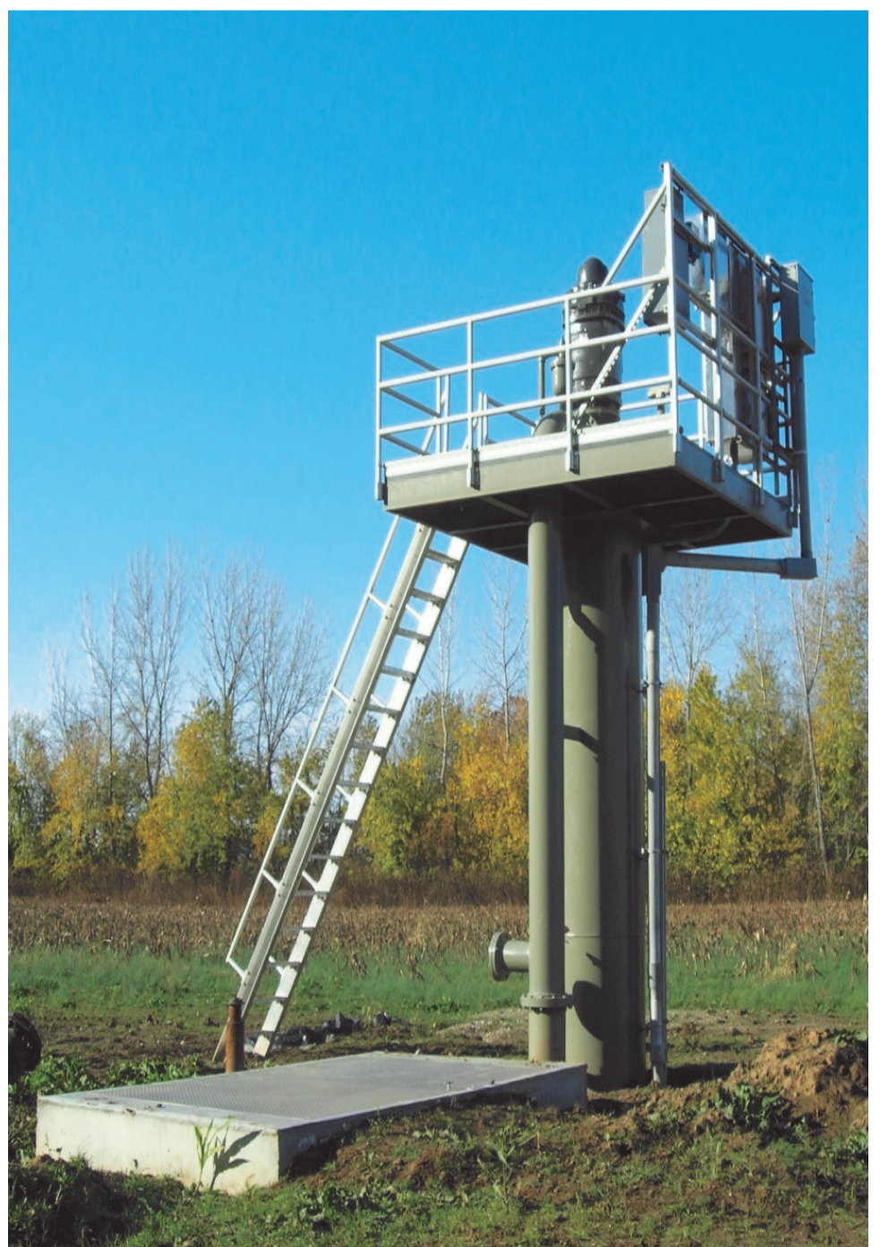
A new water supply well at the Bargersville's well field.
