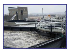
Martinsville's 1960 wastewater treatment plant was originally designed to remove Biochemical Oxygen Demand and Total Suspended Solids. On April 1, 2004, the city received a new National Pollutant Discharge Elimination System permit, which required the removal of ammonia-nitrogen at 9.5 milligrams per liter on an average monthly basis. The new permit will result in a decreased loading of ammonia, nitrogen and pathogens to the West Fork of the White River.
