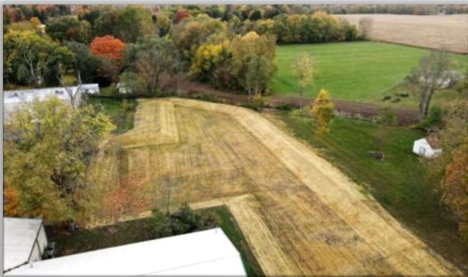
Above: Hammer Street Detention Basin
