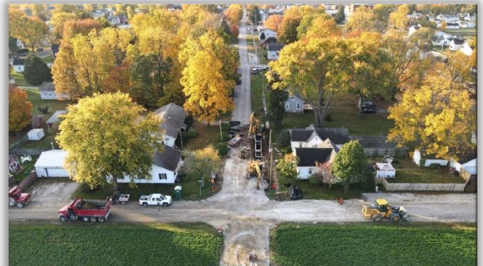
Below: Completed Storm Sewer, Line C
