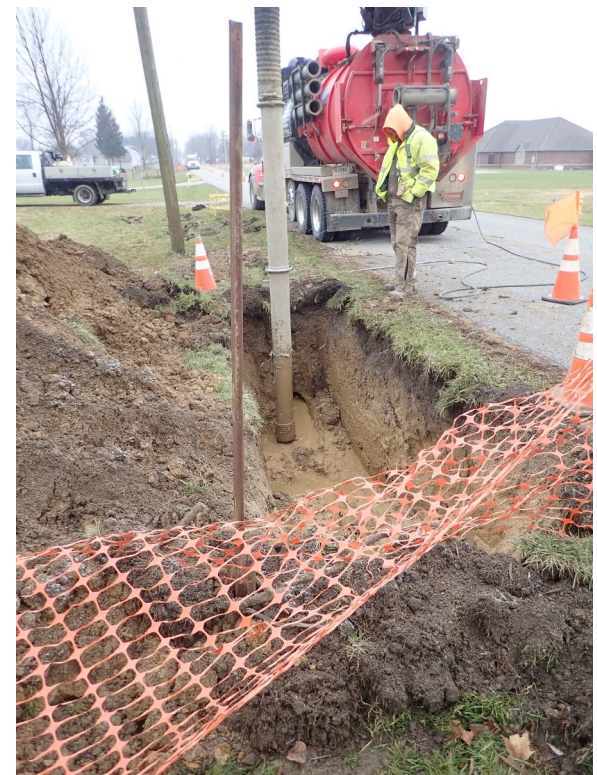
Russiaville: Pipe Installation Bore Pit
