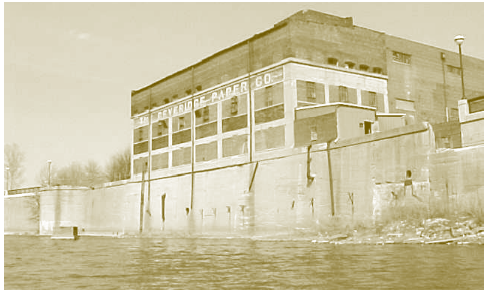
The former Beveridge Paper facility was a brownfield property that operated along the White River for more than 112 years. Demolition of the buildings began in August of 2000.
