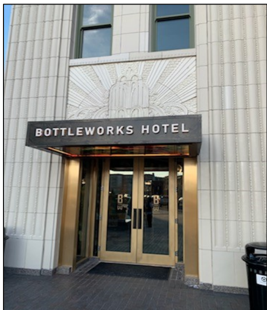
Bottleworks District Development, Indianapolis: hotel entrance
