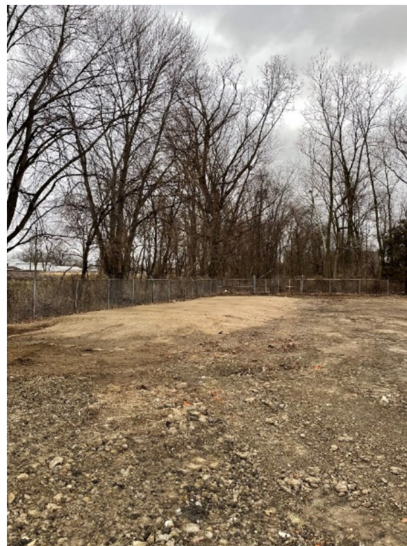
The Butler Company – Barrier 3
