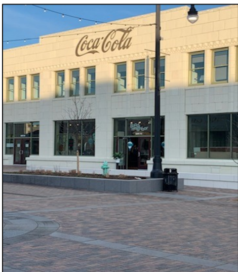
Bottleworks District Development, Indianapolis: preserved Coca-Cola art-deco style building exterior now
