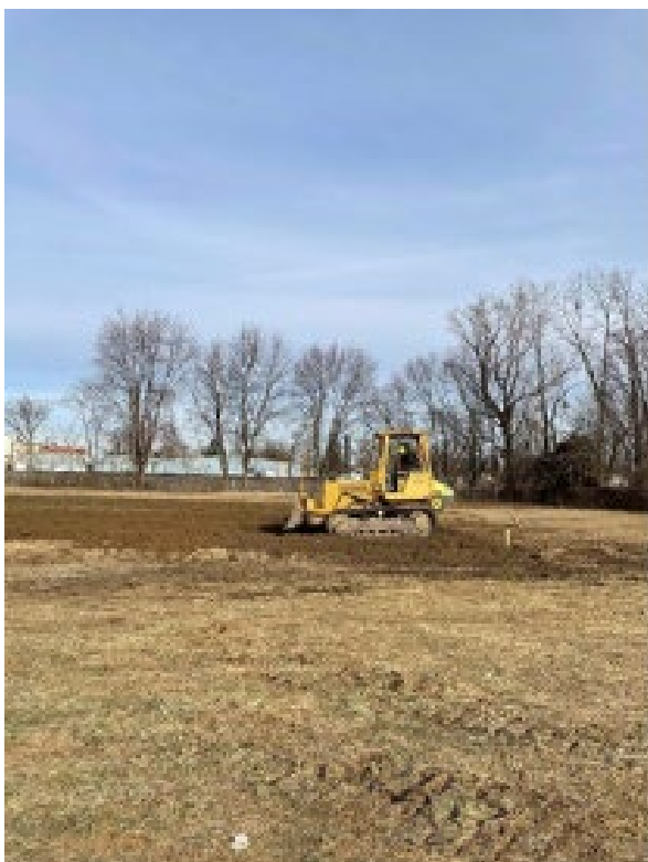
Barrier 2 under construction
