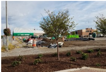
September 2019 Construction Site
