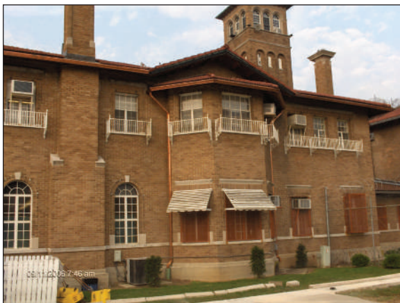
As part of the ongoing renovation of the Administration Building at the Pendleton Correctional Facility, new copper gutters were recently installed.
