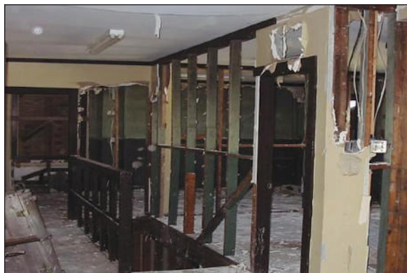
(construction of barracks during)
