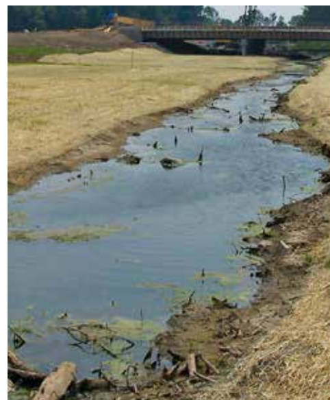
Construction within a floodway.
