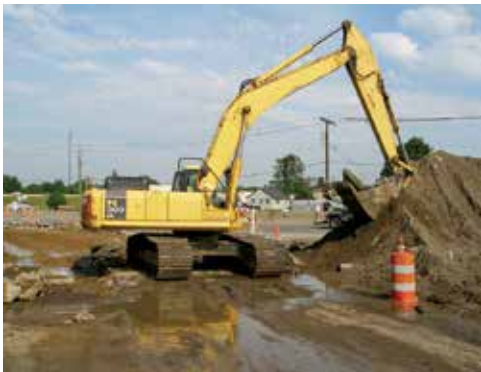
Construction activity exceeding one acre.
