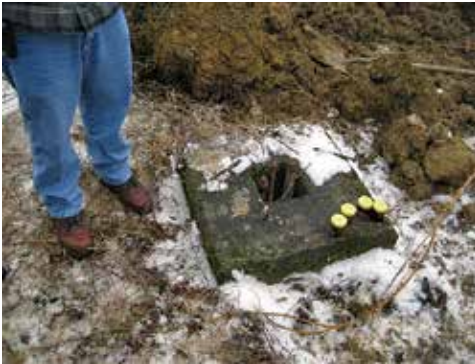
Remnants of a dispenser pad for a UST.
