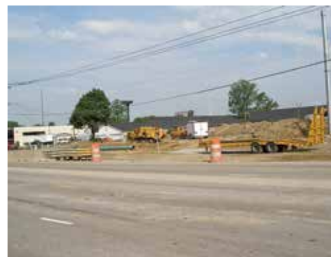
Construction activity exceeding one acre.
