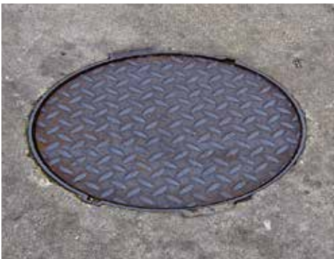
Fill pad for a UST.
