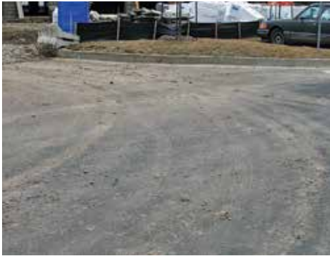
Extensive soil build-up.
