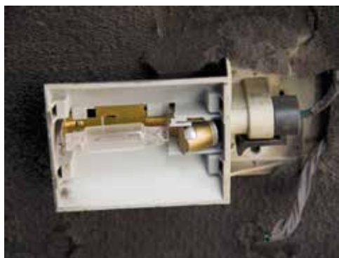
Mercury is contained within the gold-colored pellet near the right end of this mercury switch housing.
