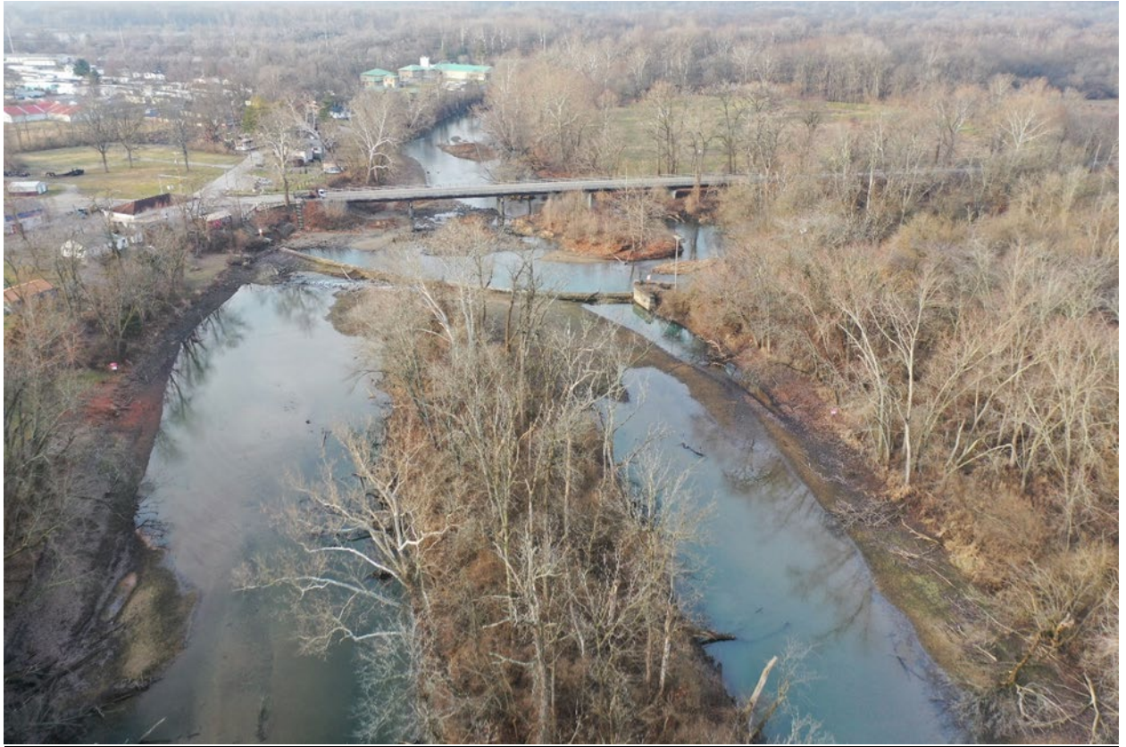
Figure 14. Drone picture from upstream of the dam looking downstream. Photo taken 8 January 2024. Thompson Mill dam, Edinburgh Indiana. Note the lower water level because as a result of the breach in the dam.
