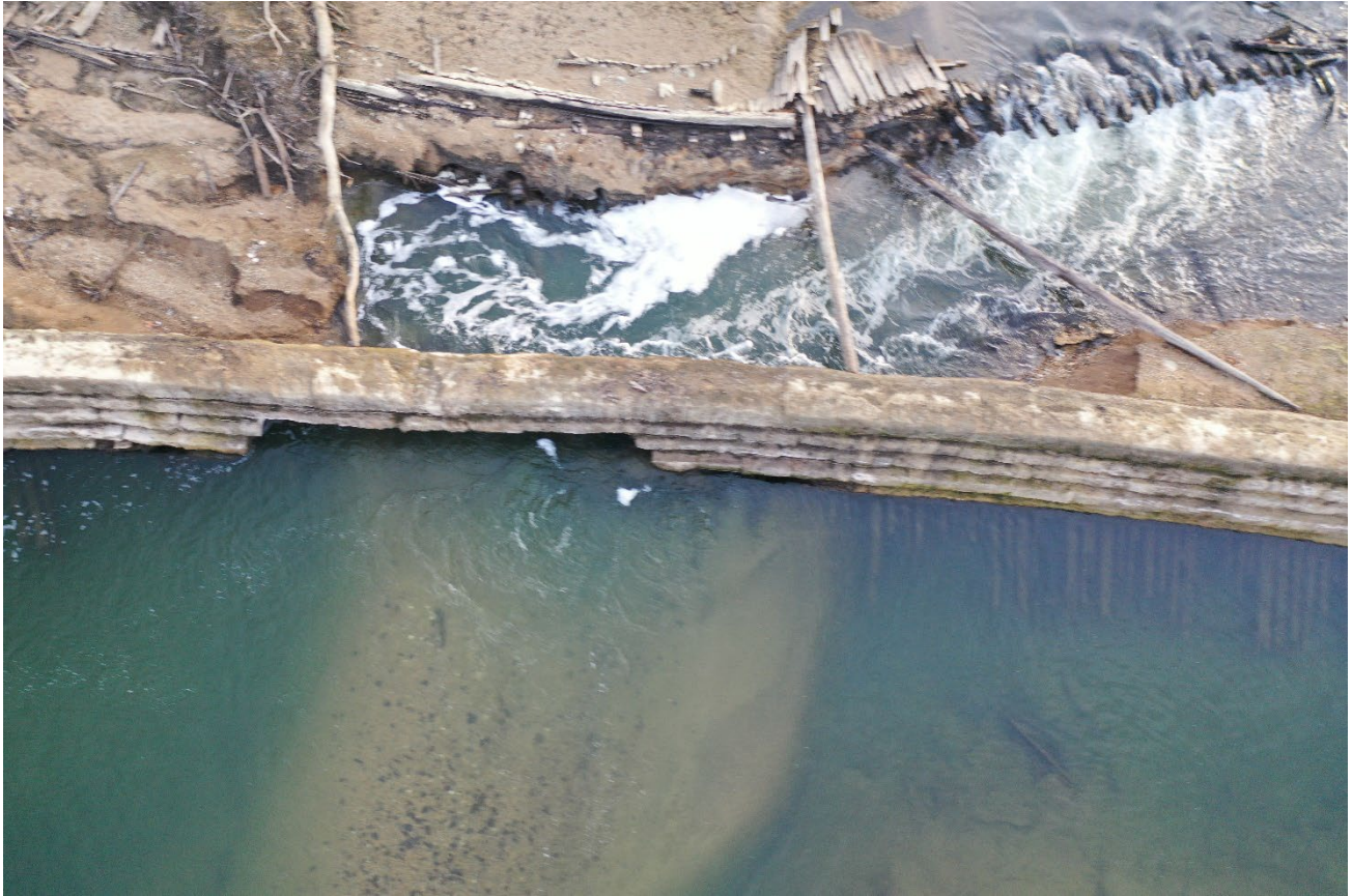
Figure 16. Breach in the Thompson Mill Dam and sediment plume. Note exposed logs on the right side of the image.
