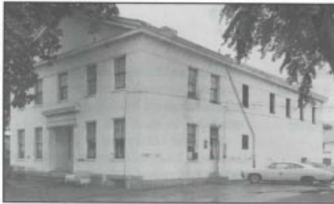
This Jefferson County jail and sheriff's residence was accepted by the County Commissioners in 1849. It is built of brick and stone and is an example of the Greek Revival style of architecture in the mid-nineteenth century. The vacated structure still stands in Madison, and self-guided tours are available. The photograph was taken circa 1965.
