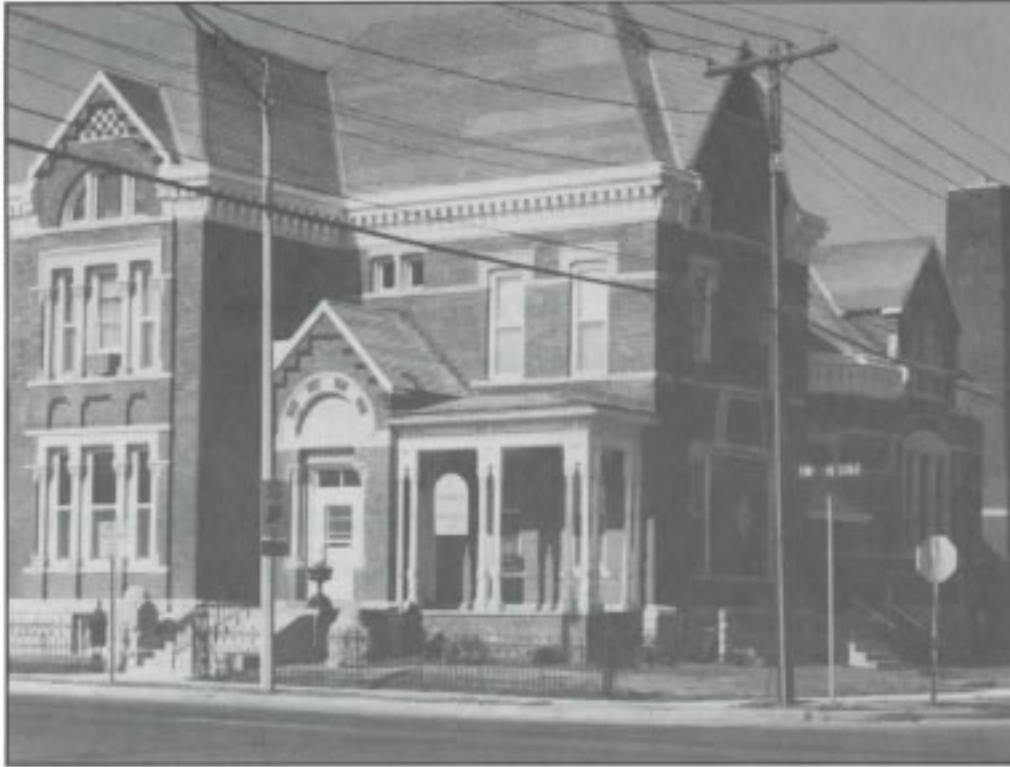
This photograph of the 1882 Montgomery County jail and sheriff's residence in Crawfordsville was taken circa 1988 after remodeling as the Old Jail Museum. The jail structure is behind the residence.
