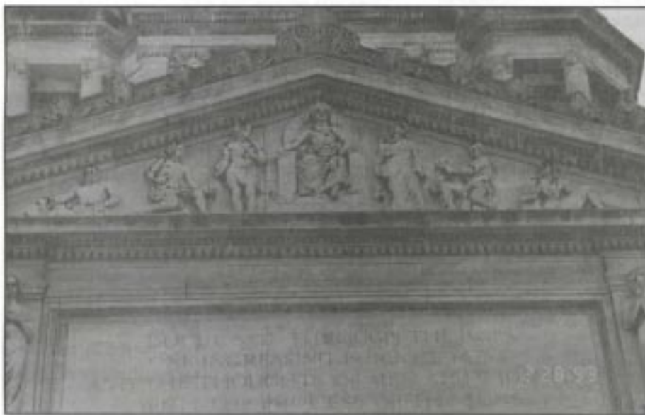
6. Each side of the Allen County Courthouse has a similar sculptural element. The Renaissance-style courthouse, made from limestone, was dedicated September 23, 1902.
