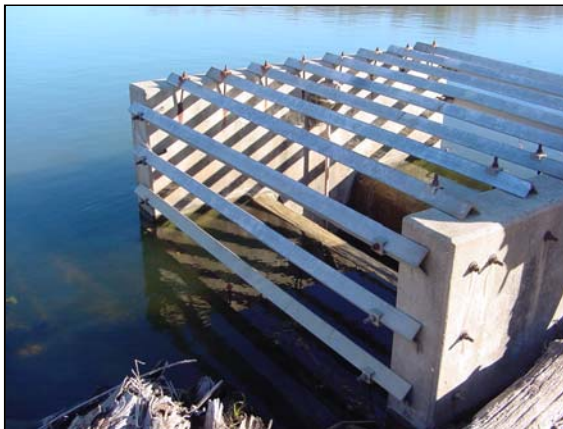
Figure 3 – Trash rack design with fish protector screen
