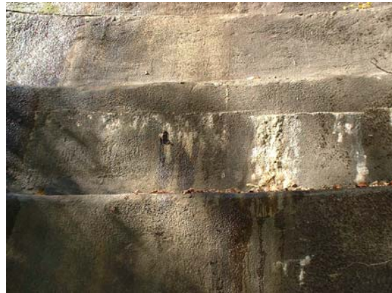
Figure 3 – Efflorescence
