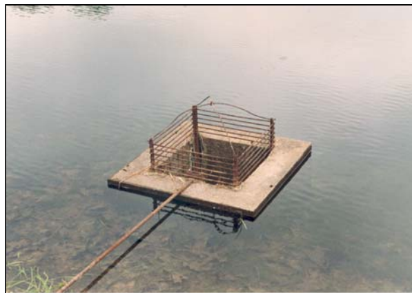
Figure 4 – Examples of trash racks used in Indiana
