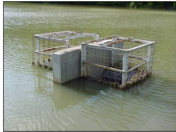
Figure 3 – Trash rack design with fish protector screen
