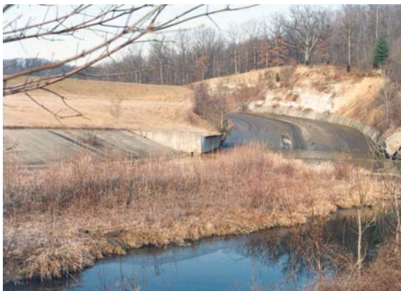
Figure 1 – Concrete chute spillway
