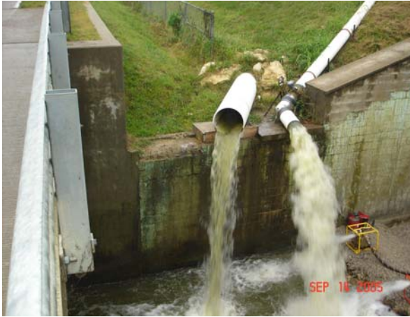
Figure 2 – Lake drain consisting of a pipe with control valve (left) and a siphon drain (right).
