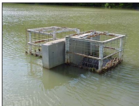
Figure 2-7 Trash racks on riser spillway structure.
