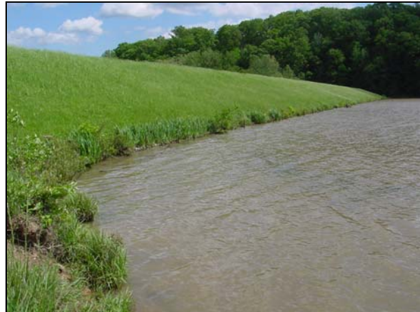
Figure 2-1 Earth embankment dam in Indiana.
