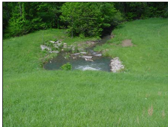
Figure 2-5 Riprap-lined stilling basin at spillway outlet.
