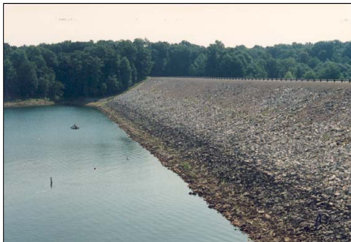
Figure 2-11 Riprap slope protection on an embankment dam.
