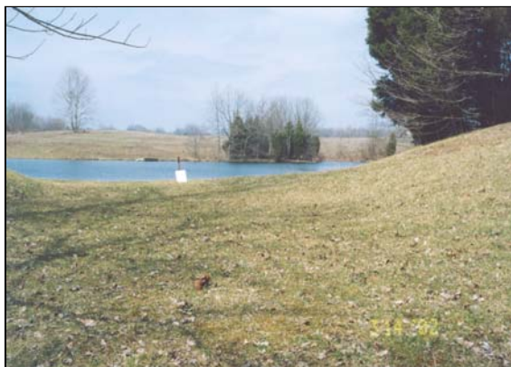
Figure 2-10 Grass-lined emergency spillway.
