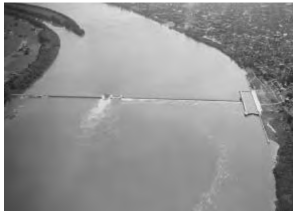
River bends at the old lock and dam 46, one of the old wicket dams at Owensboro, Kentucky (ca. 1930). (All images on this page are courtesy U. S. Army Corps of Engineers)
