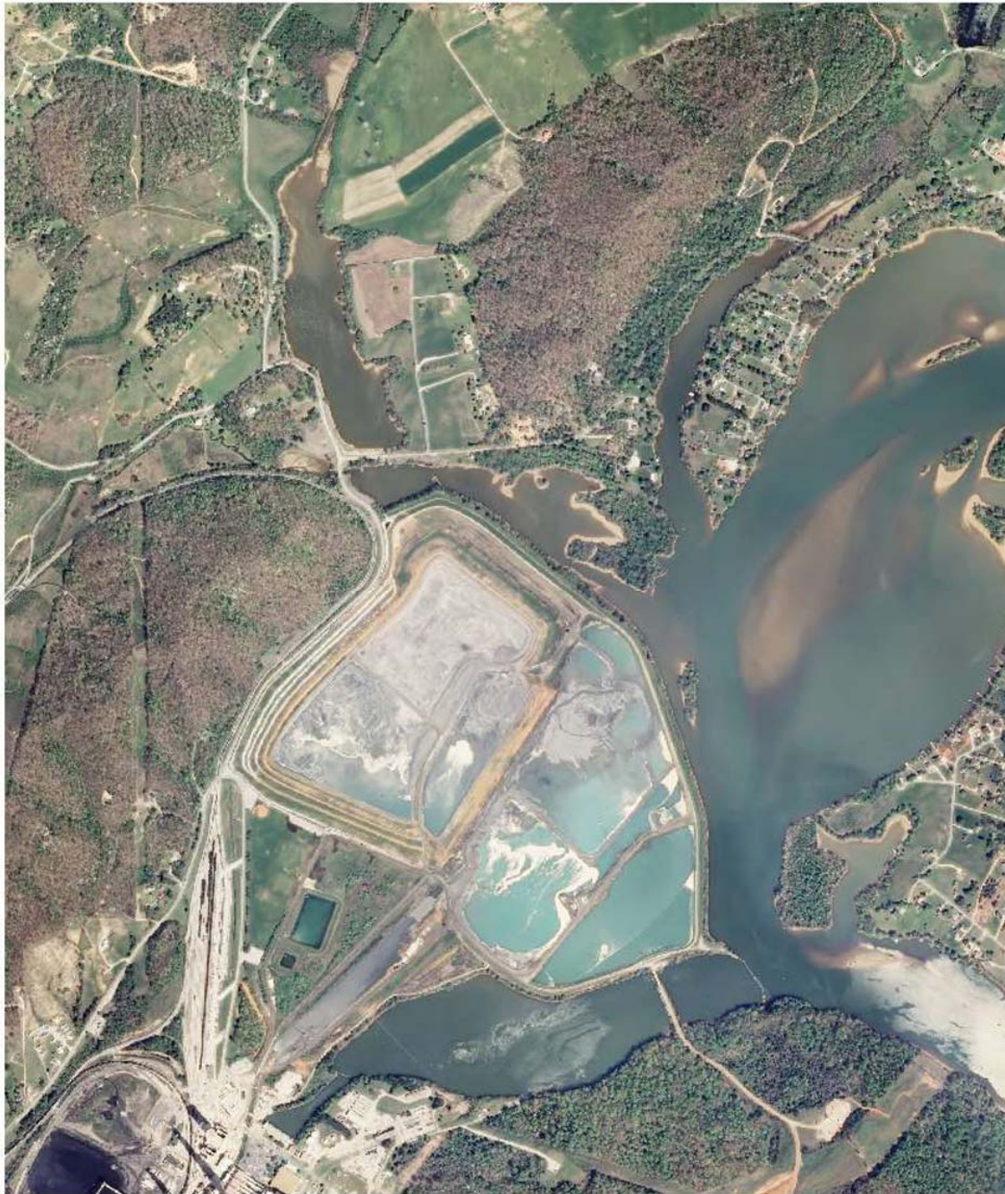
Aerial Image of Kingston Ash Slide Pre-Event 2008
