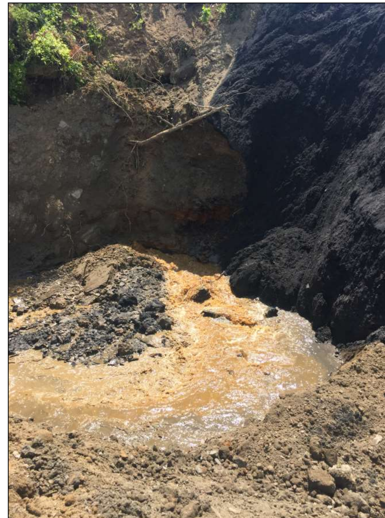
Dewatering efforts caused blowouts due to the volume of the mine pool.
