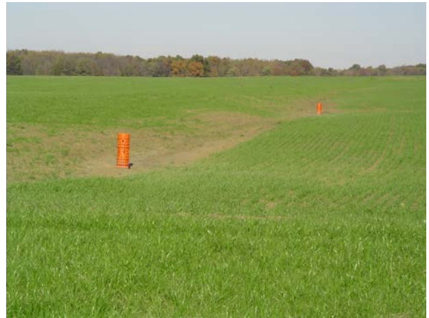
Water control structures on recently reclaimed land. These include grass waterways (bottom left), WASCObS (upper and lower left). Photos courtesy of Peabody Coal.
