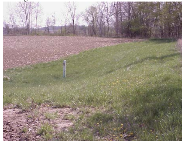
WASCOB embankment (right) and riser for drainage
