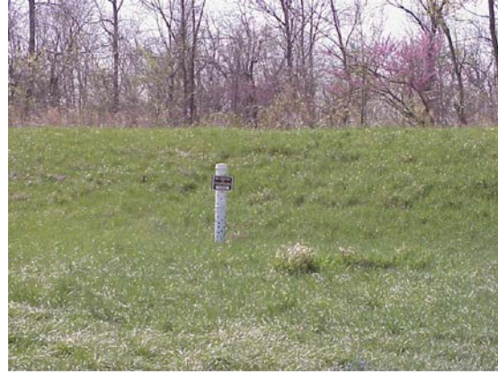
WASCOB embankment (behind riser) and riser for drainage
