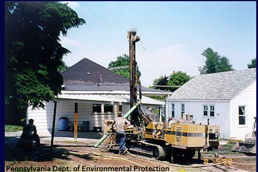
Mine void grouting
