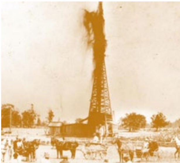
Old Trenton well drilled in the late 1800s
