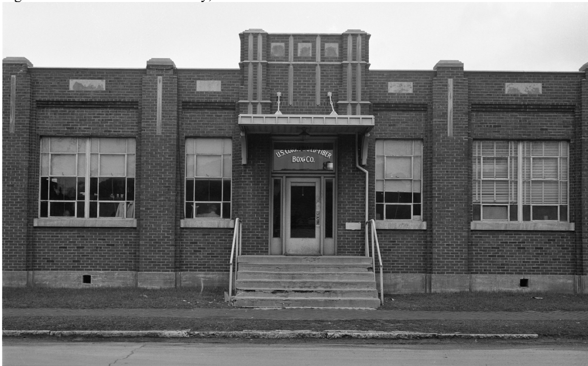
Figure 10: The primary north-facing elevation of Building E, displaying Art-Deco ornamentation
