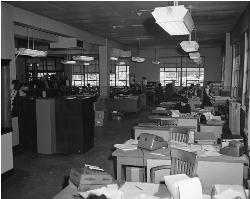
Figure 14: Interior of the offices located in Corrugated-Fibre Plant Building E
