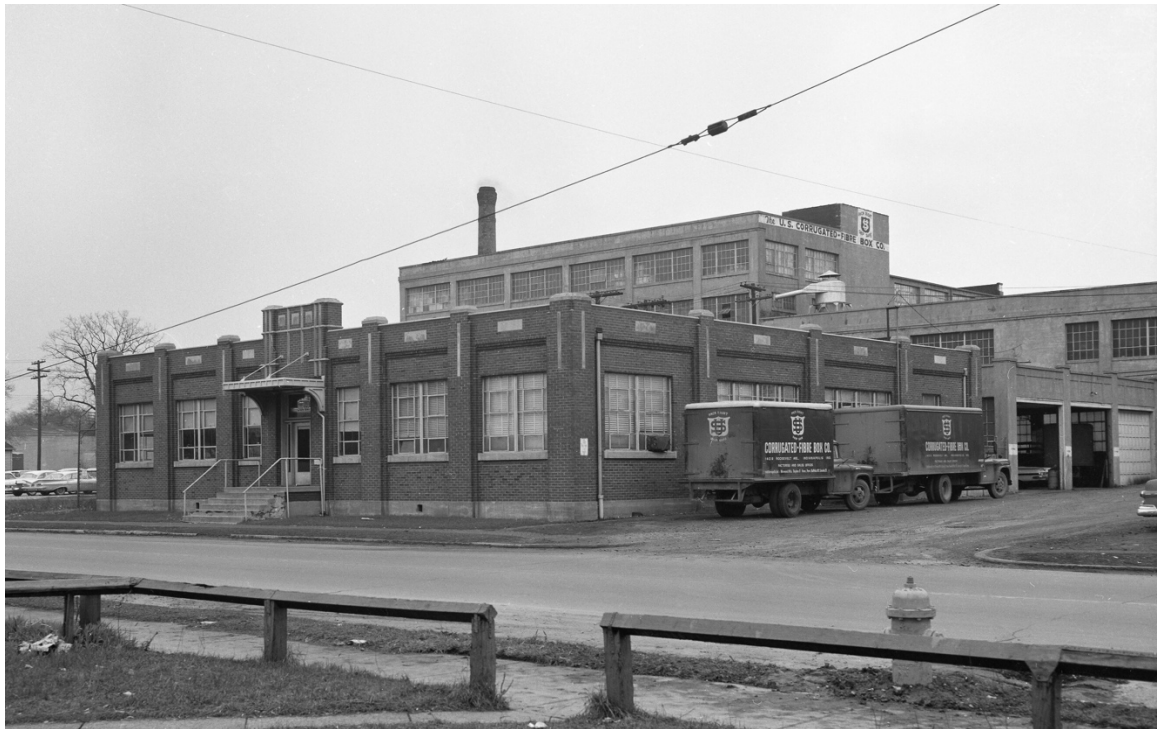
Figure 12: The Corrugated-Fibre Plant, facing southeast, date unknown
