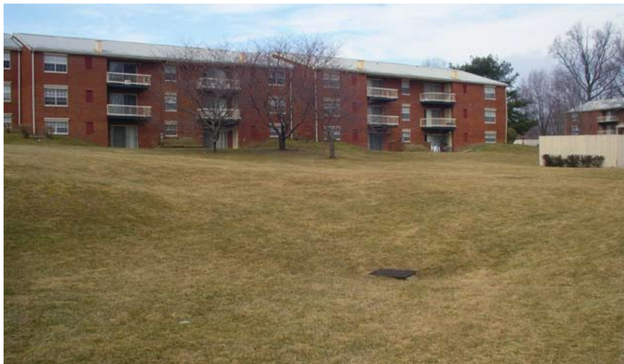
Figure 9. This at-capacity site receives rooftop runoff from adjacent townhomes.
