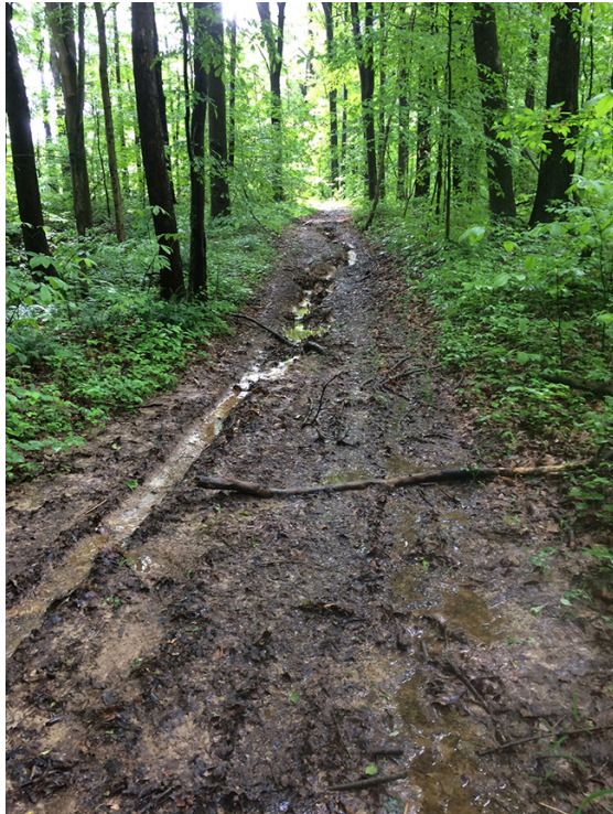
LEFT: Skid trail with gully erosion due to lack of water diversions. RIGHT: Water-bar outlet conveying runoff on to the stable forest floor. Photos by Duane McCoy, DNR
