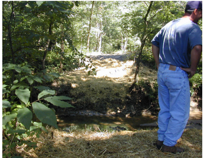
TOP LEFT: On a private site: No water diversions before stream crossing. No stream bank stabilization/revegetation. TOP RIGHT: A skidder crosses a log bridge. BOTTOM LEFT: Dozer installing bridge for stream crossing during a demonstration. BOTTOM RIGHT: A well closed-out stream crossing, with seed and straw applied to stabilize bare soil and promote revegetation. All Photos by Duane McCoy, DNR
