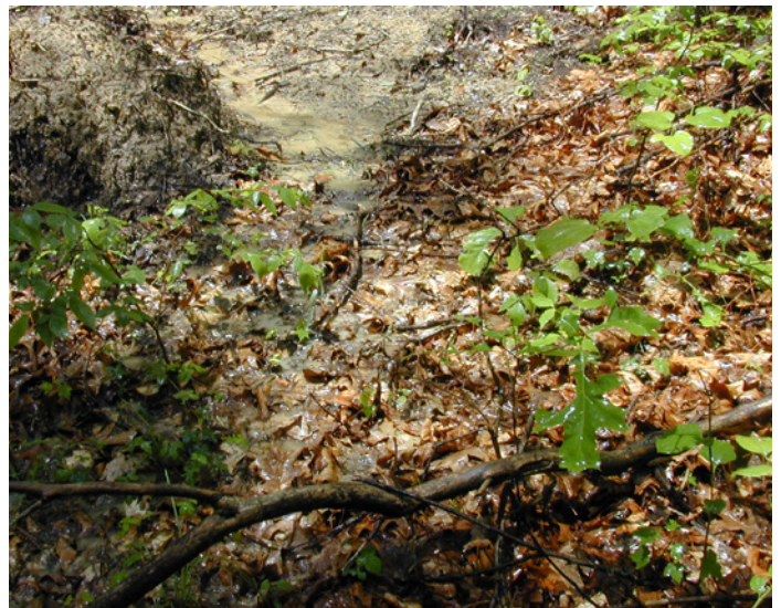
Water-bar outlet conveying runoff on to the stable forest floor. Photo by Duane McCoy, DNR
