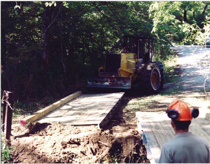
TOP LEFT: On a private site: No water diversions before stream crossing. No stream bank stabilization/revegetation. TOP RIGHT: A skidder crosses a log bridge. BOTTOM LEFT: Dozer installing bridge for stream crossing during a demonstration. BOTTOM RIGHT: A well closed-out stream crossing, with seed and straw applied to stabilize bare soil and promote revegetation. All Photos by Duane McCoy, DNR
