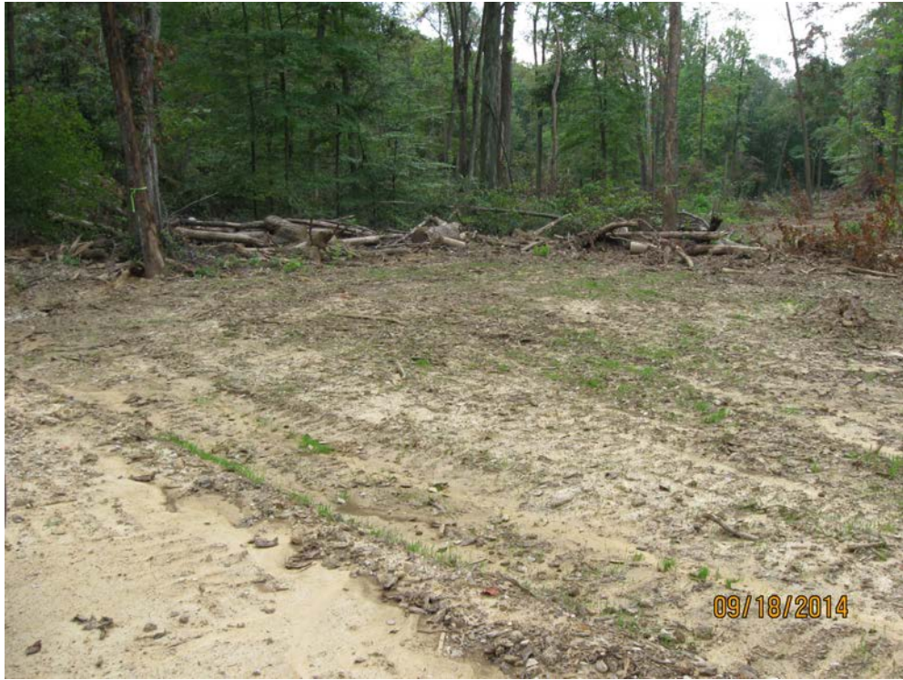
Log landing recently closed out with grass sprouting from seeding.
