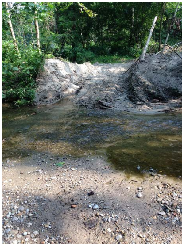
A poorly applied and implemented stream crossing with no attempt to repair. There are no water diversions before stream crossing, no stream bank stabilization/revegetation.
