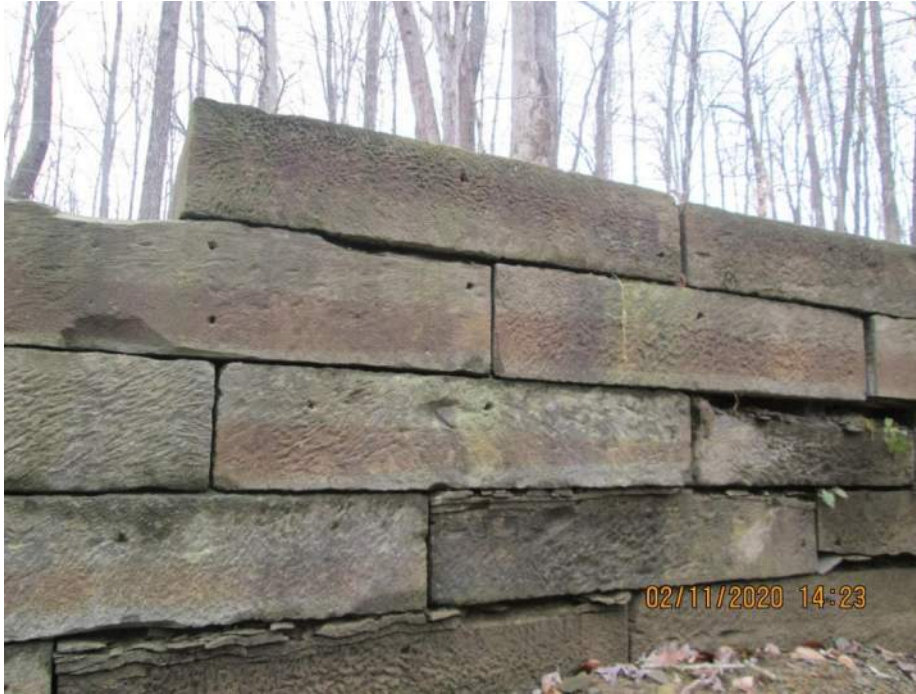
10+75 to 11+00 Delamination
