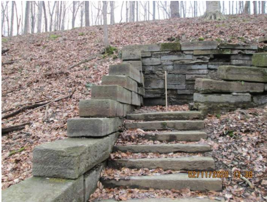
10+05 to 10+28 Landing and Bend - Landing Stone Missing Isolated Delamination - Wall wedged over Walkway
