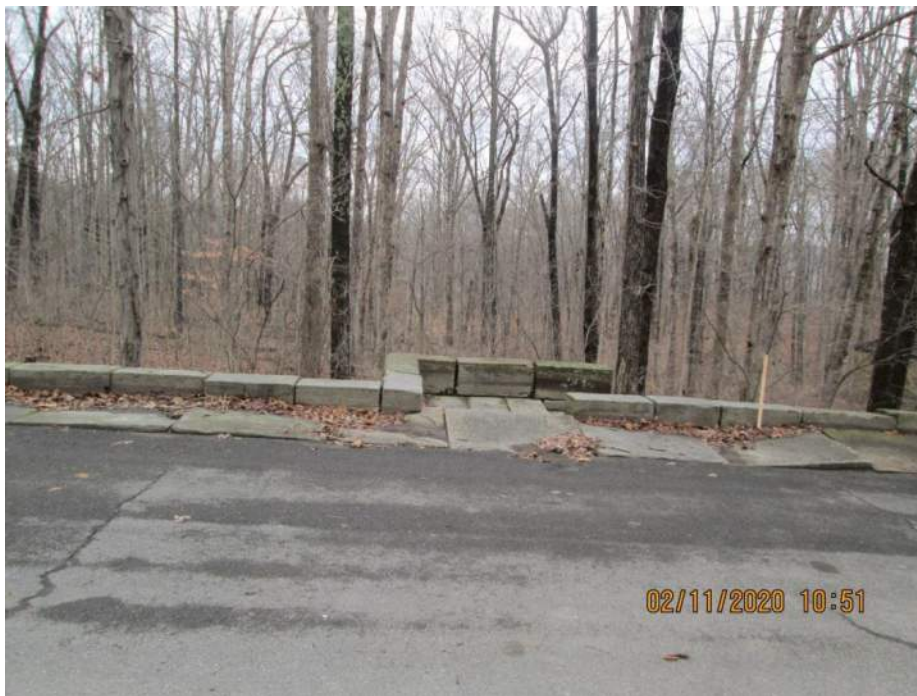
12+25 to 12+50 Block separation Stairs
