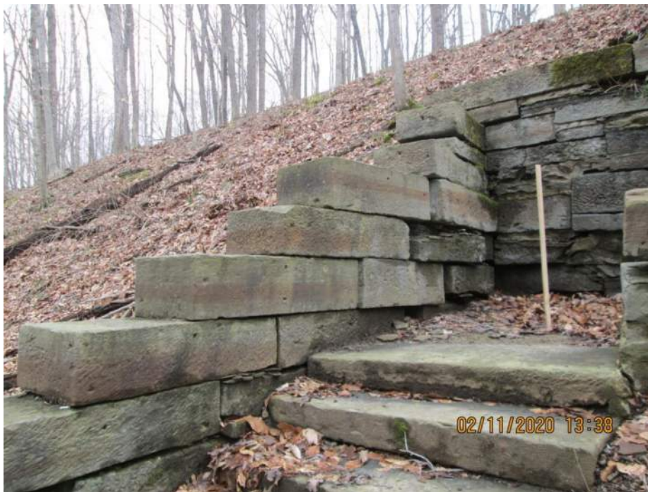
10+05 to 10+28 Landing and Bend - Landing Stone Missing Isolated Delamination - Wall wedged over Walkway
