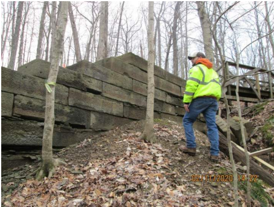
10+75 to 11+00 Delamination
