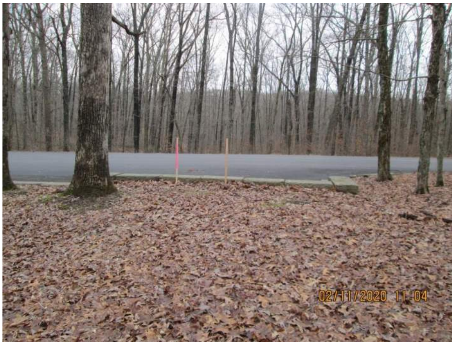
10+30 Wall at Grade -
