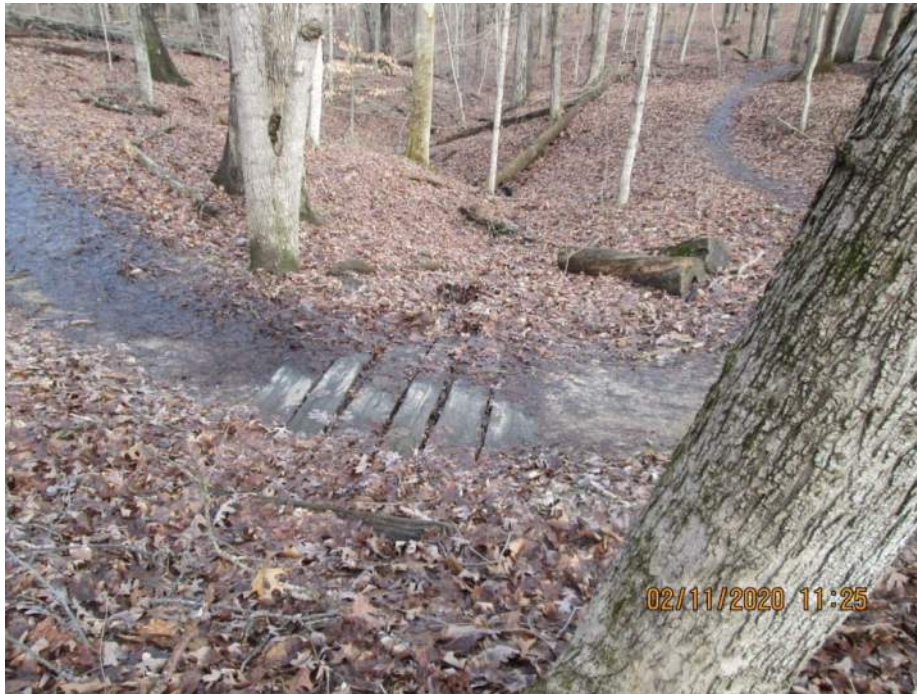
12+75 Detail Drainageway at 12+75 following foot path to North
