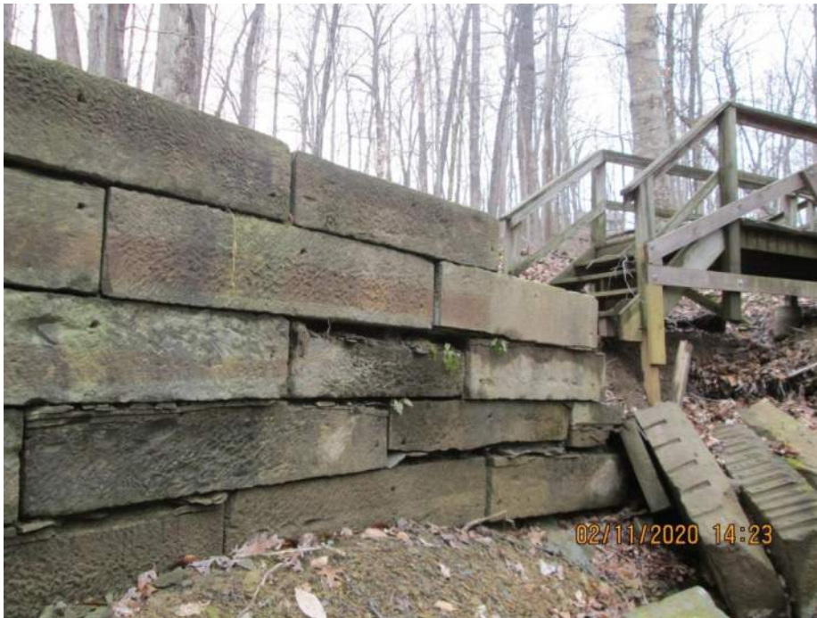
10+75 to 11+00 Delamination
