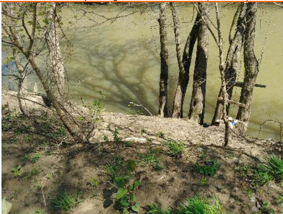
Photo 8: Slope along Indian Kentuck Creek (East)
