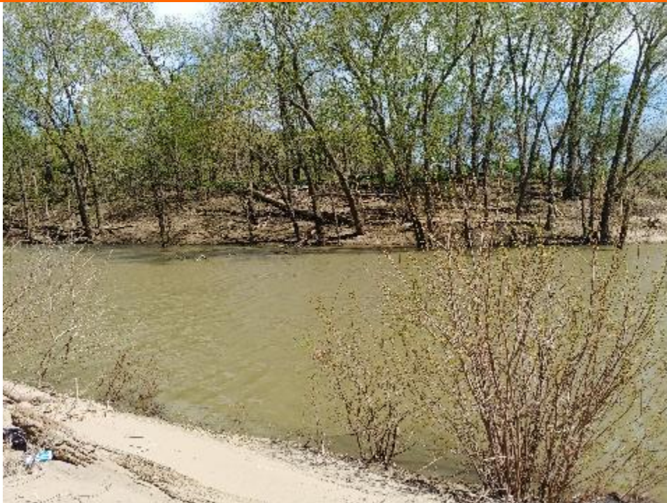
Photo 6: Slope along Indian Kentuck Creek (East)
