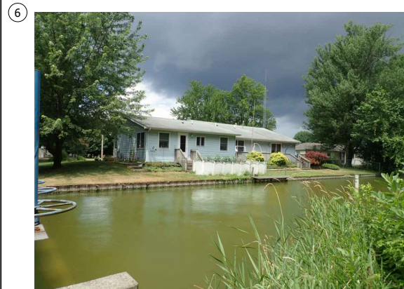
EXISTING UPSTREAM SHEET PILING
