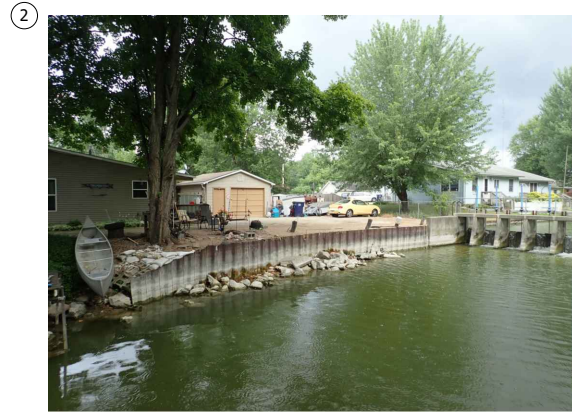
EXISTING DOWNSTREAM SHEET PILING
