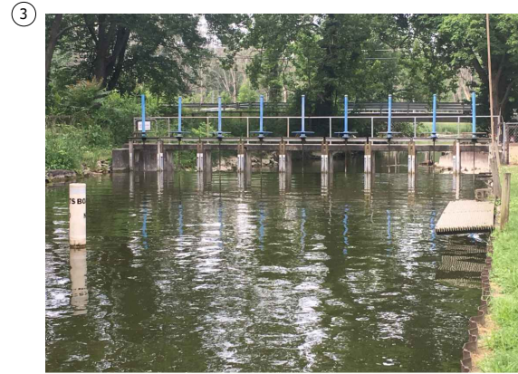
EXISTING OUTLET STRUCTURE LOOKING DOWNSTREAM
