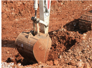
Digging projects that begin before calling 811 can result in hitting a utility line, causing outages or injuries and repair costs.
