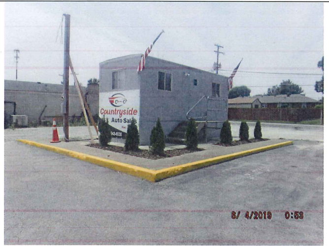
Temporary Building Looking to West
