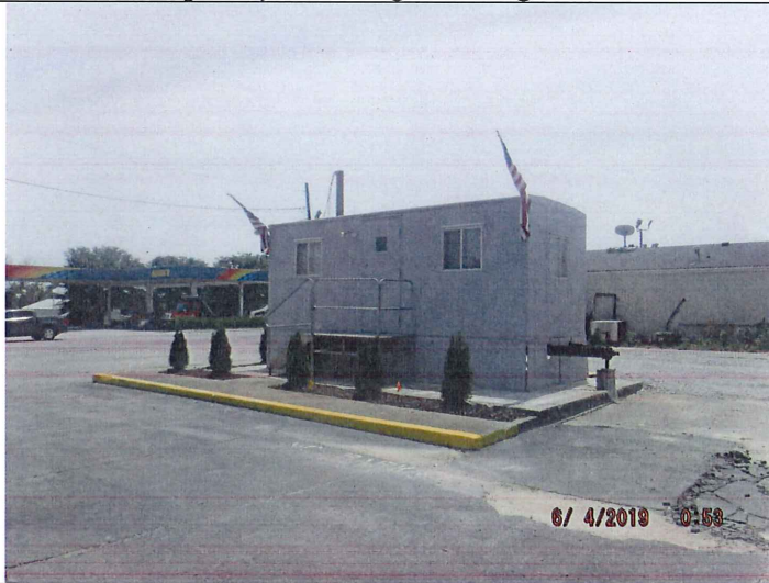
Temporary Building Looking to South
