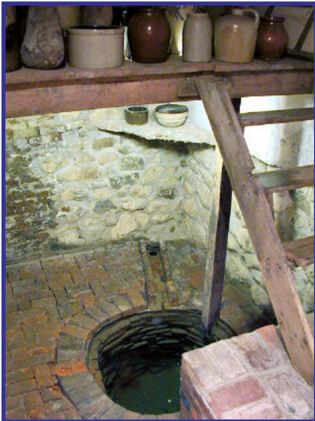
Hidden indoor well in basement
