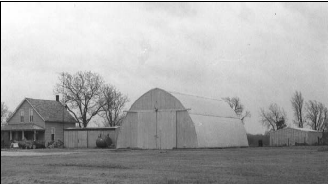
Grade C Quonset
