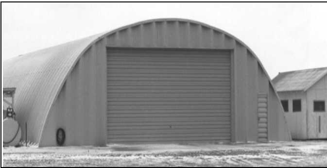
Grade C Quonset
