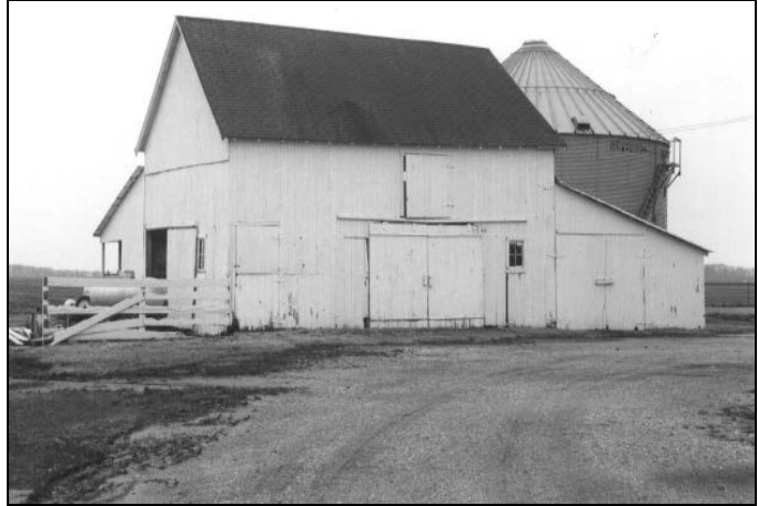
Average Condition Foundation-Solid Walls-Sound Structure-Sound Roof-Sound
