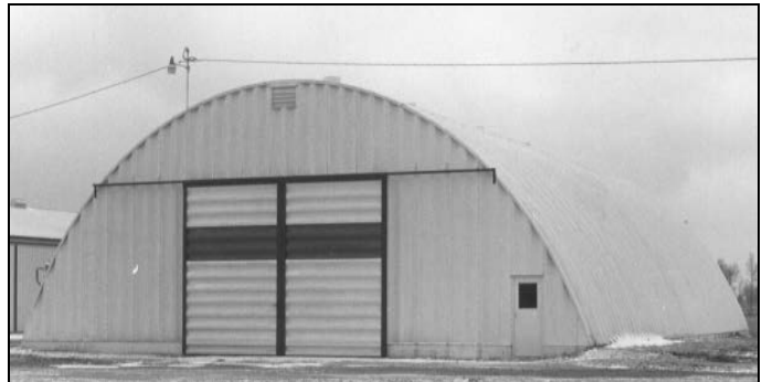
Grade C Quonset
