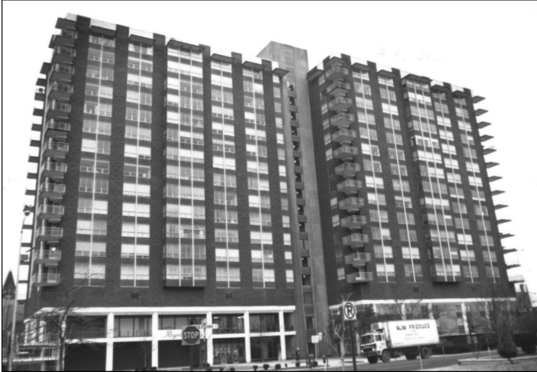
Grade C Apartment Building
