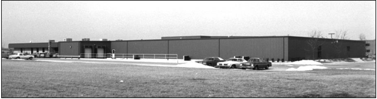
Grade C Light Industrial Facility
