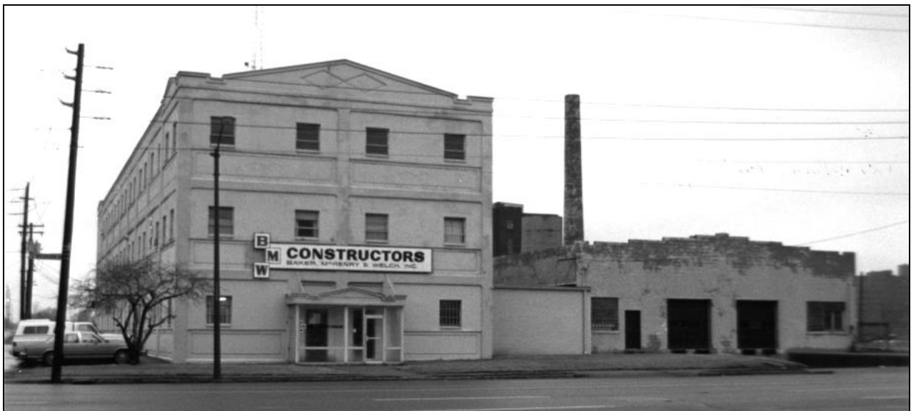
Grade C Loft Industrial Facility
