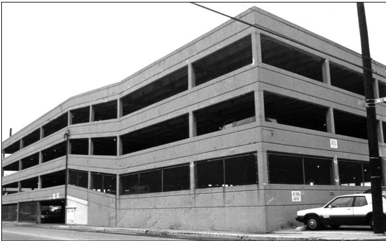
Grade C Parking Garage
