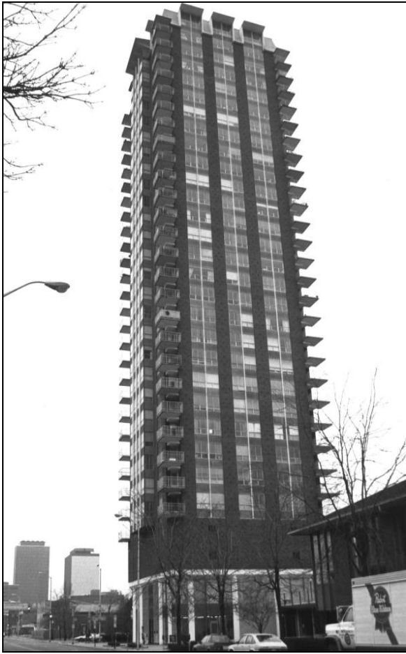
Grade C Apartment Building
