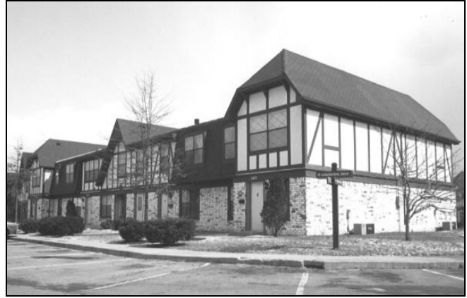
Grade C Apartment Building
