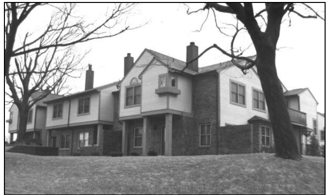
Grade C GCR Apt. Building or Res. Schedule A (depending on design)
