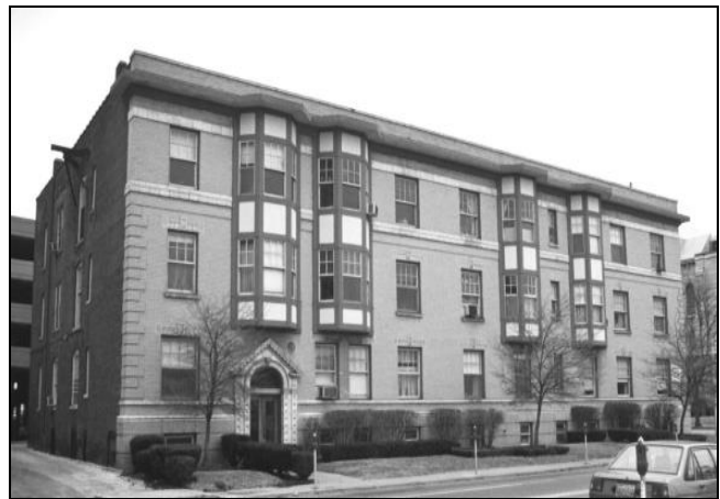
Grade C Apartment Building
