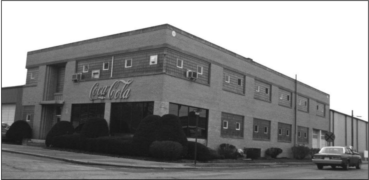
Grade C Loft Industrial Facility
