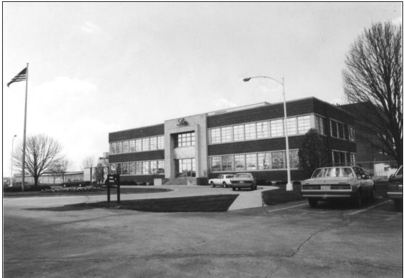
Grade B Industrial Office
