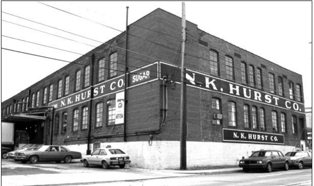
Grade C Loft Industrial Facility
