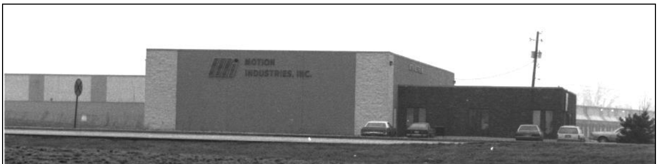
Grade C Light Industrial Facility
