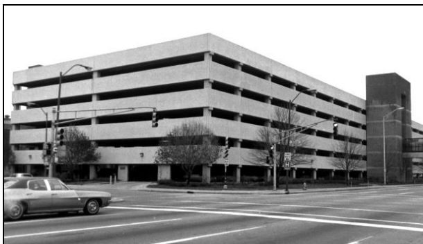
Grade C Parking Garage
