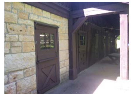
CCC-built Nature Center
