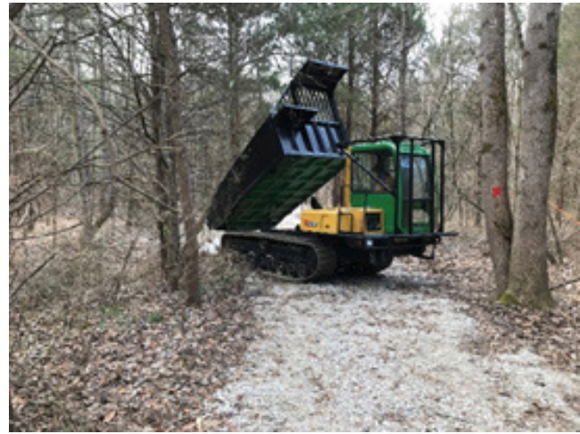
DNR trail crew utilizing specialized equipment
