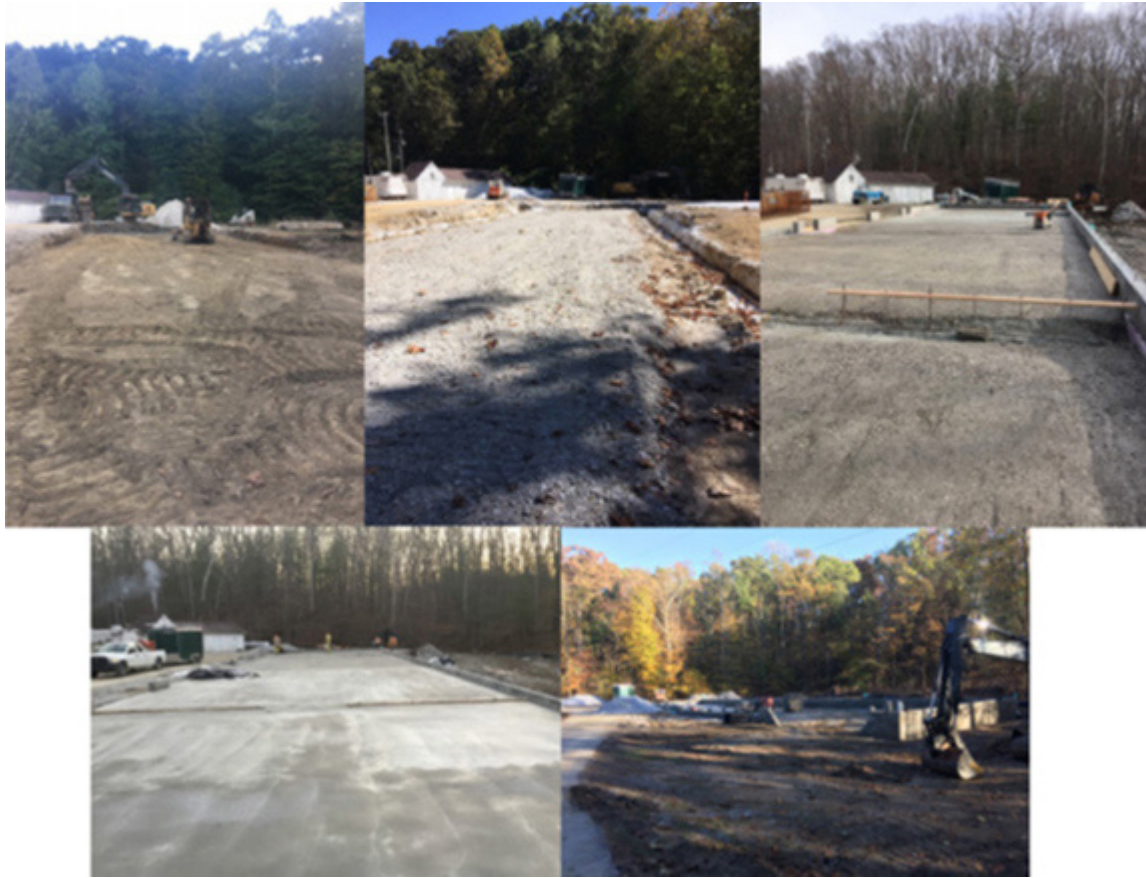
Figure 3. Jackson-Washington State Forest 7-bay garage and storage building.
