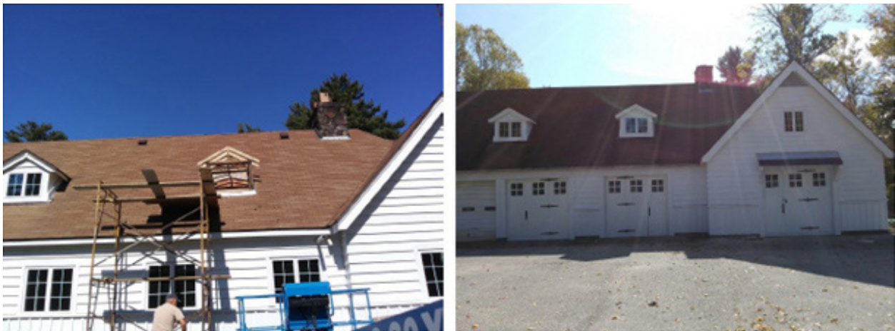
Figure 1. Ferdinand-Pike State Forest exterior renovations.
