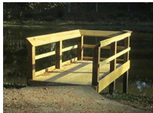
Figure 7. Renovated fishing pier at Clark SF.
