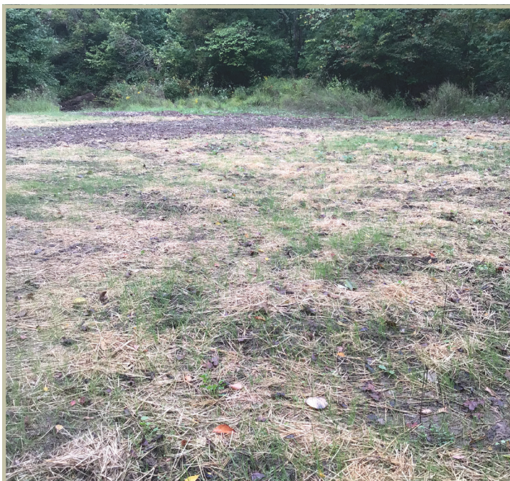
A well-closed-out log landing, smoothed, strawed, and seeded. Photo by Duane McCoy.
