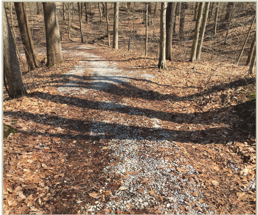
Stable access road with rock and water diversions.
