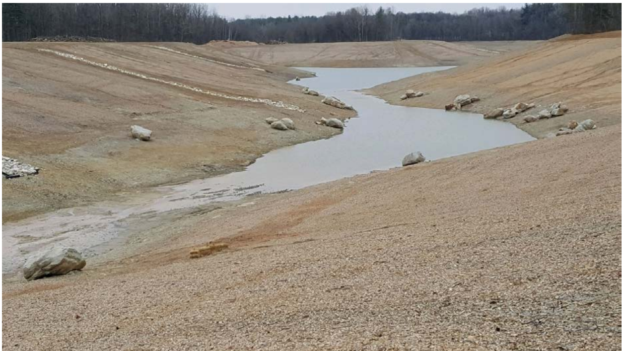
The Gambill Lake restoration at Greene-Sullivan State Forest was done in cooperation with the DNR Division of Reclamation to address dangerous highwall conditions from mining activity done the mid-1900s.
