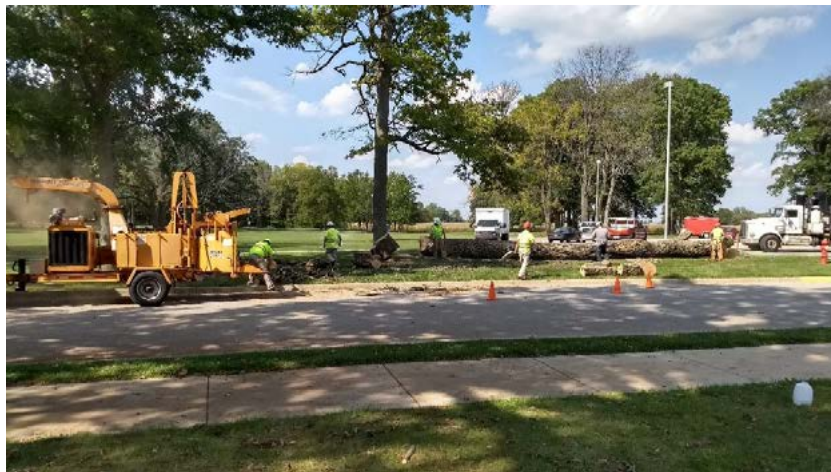
Large dead ash removed from along the main road at the Indiana Veterans' Home.
