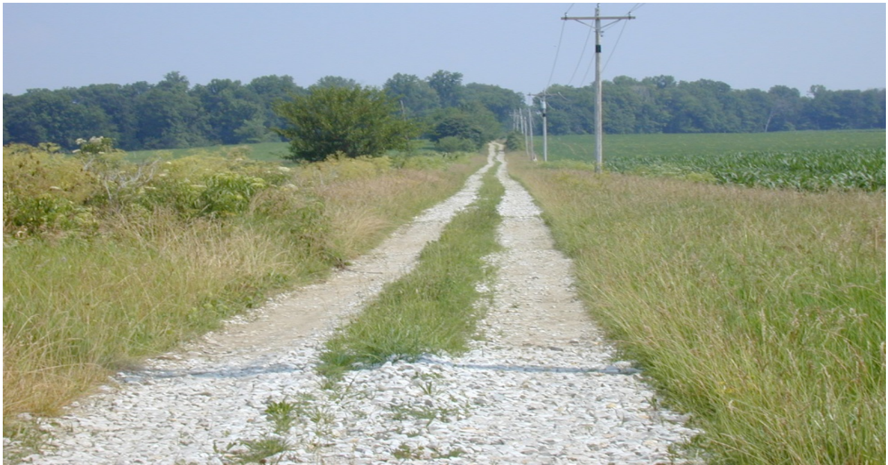
Permanent haul road protected by rock.
