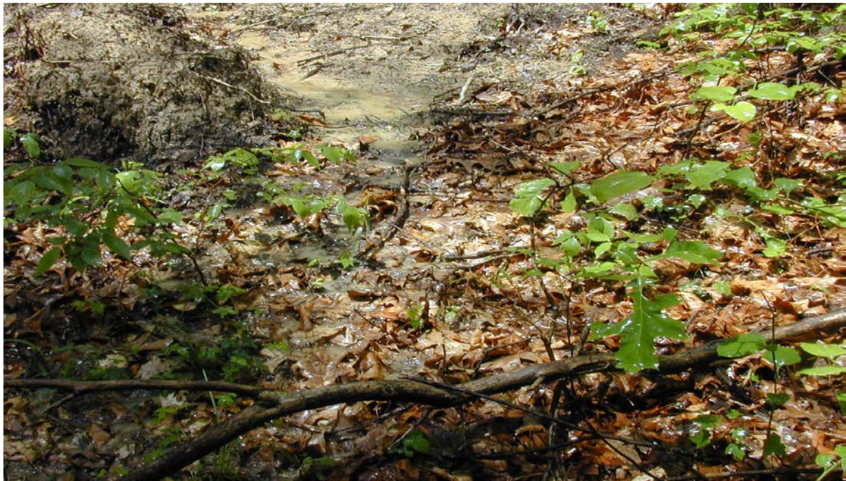
Water bar outlet conveying runoff On to the stable forest floor.
