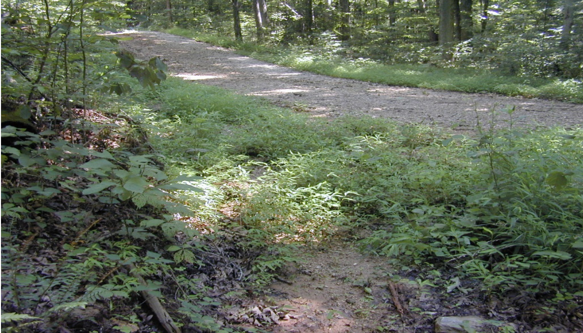
Effective cut out on a permanent access road.
