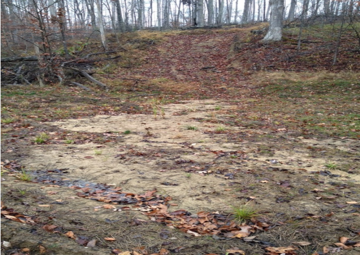
Skid trail not closed out, causing erosion and sediment plume to build up on log yard.
