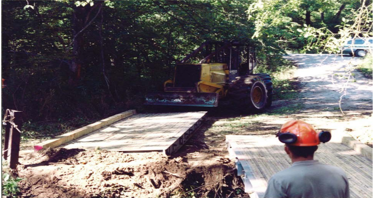
Dozer installing bridge for stream crossing on timber-harvest site.
