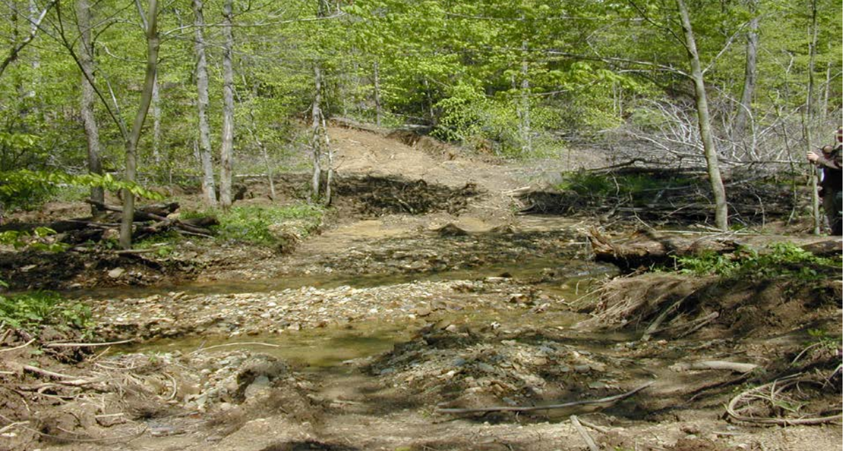
A stream crossing that was poorly executed and not closed after the harvest was completed.
