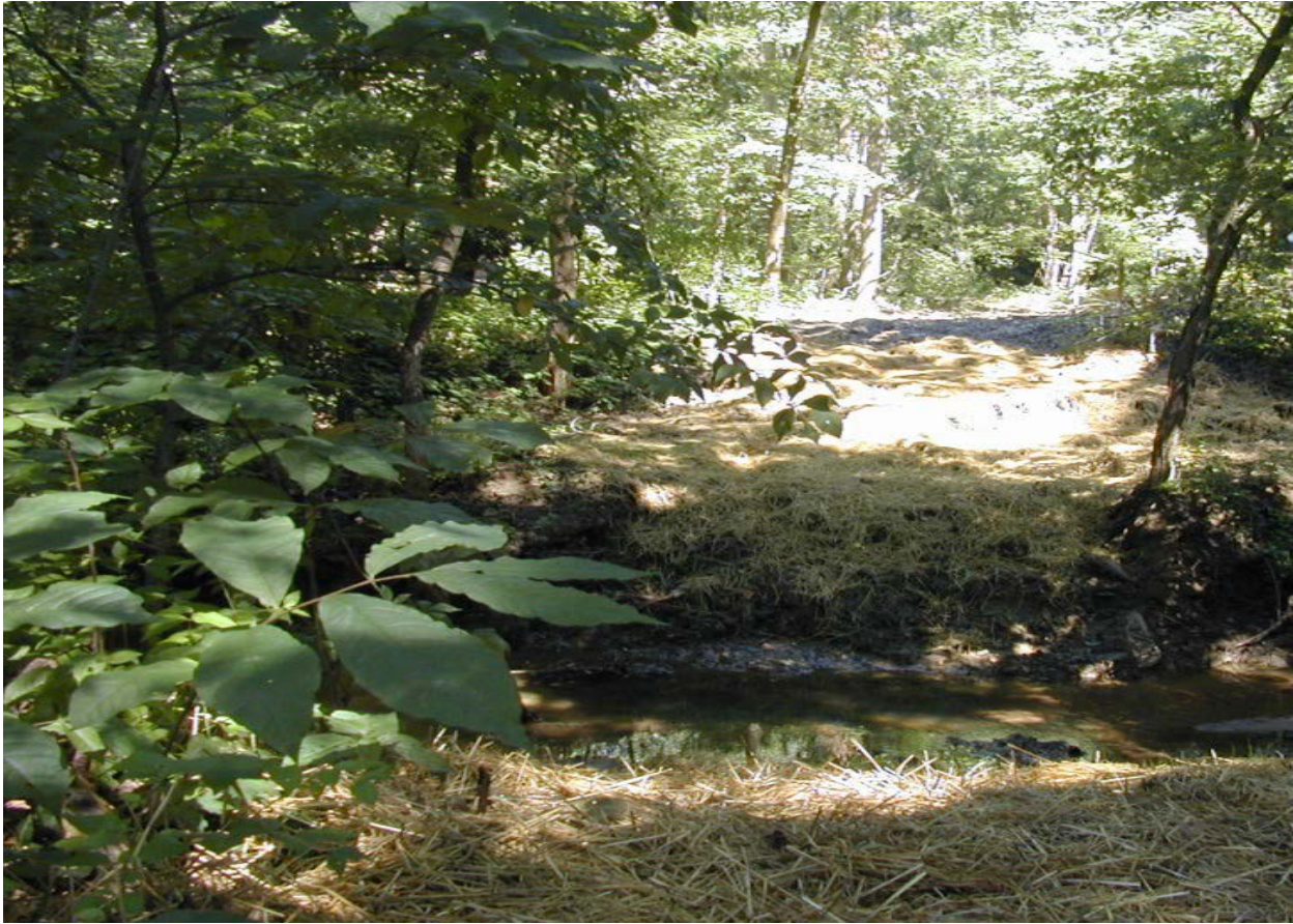
A well-closed stream crossing, with seed and straw applied to stabilize bare soil and promote revegetation.
