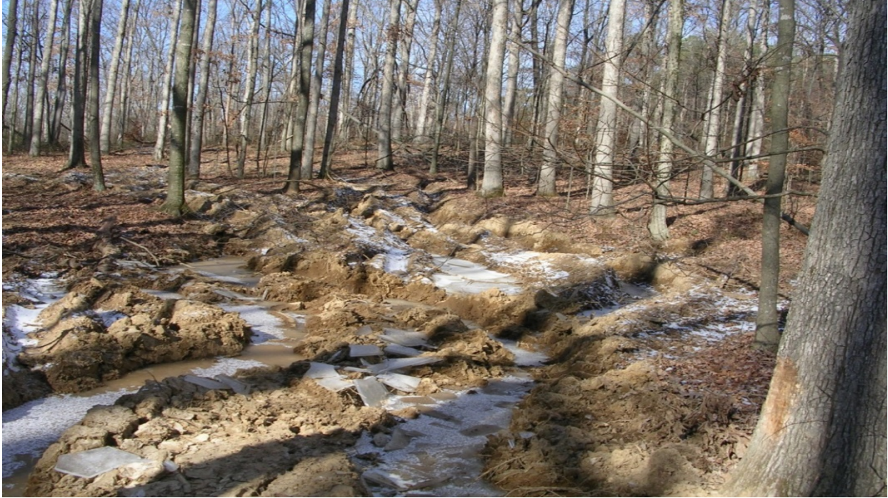
Extreme skid trail rutting due to operations taking place during wet winter conditions.
