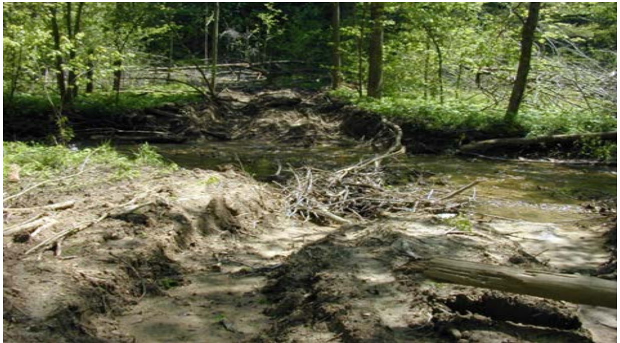
A poorly applied and implemented stream crossing with no attempt to repair. There are no water diversions before stream crossing, no stream bank stabilization/revegetation.
