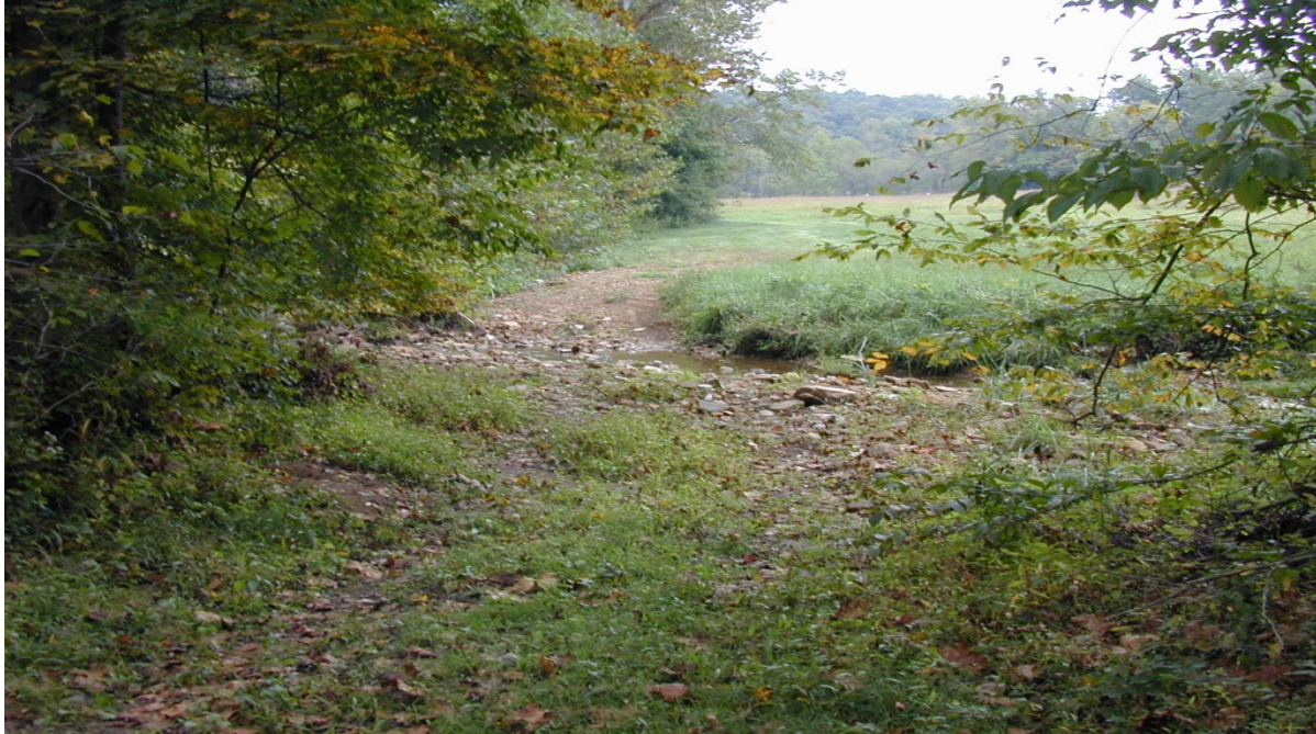
An access-road ford across a small stream with low and stable banks.
