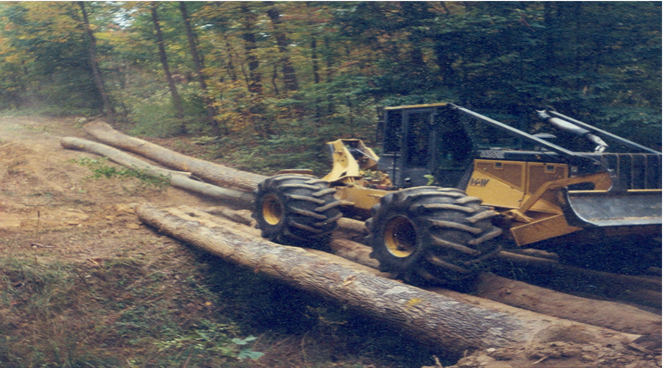
A skidder crosses a log bridge.
