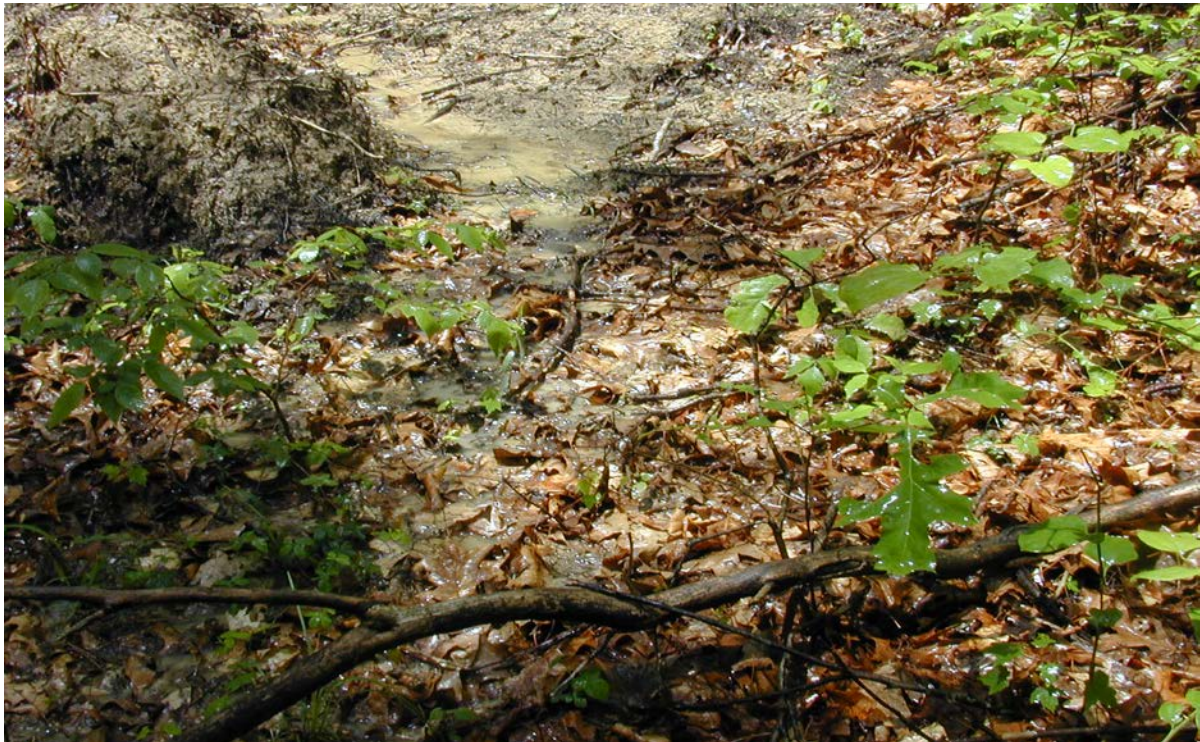
Water-bar outlet conveying runoff on to the stable forest floor.
