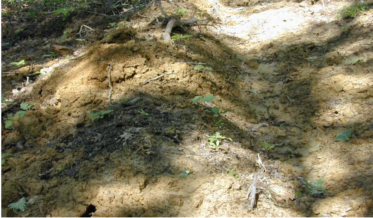
An effective water bar conveying runoff from a skid trail and diverting the flow onto the forest duff layer, where water will infiltrate the soil, the sediment will be filtered and the water will become groundwater.
