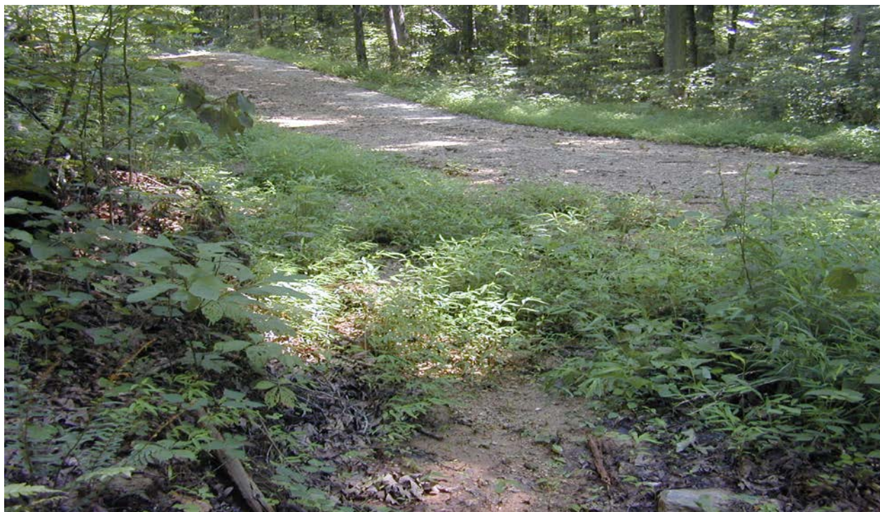
Effective cutout on a permanent access road.
