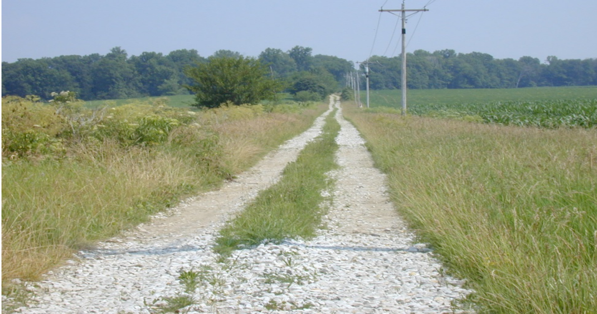
Permanent haul road protected by rock.
