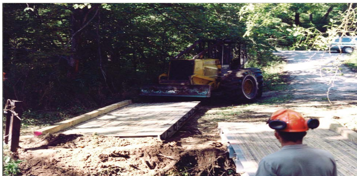
Dozer installing bridge for stream crossing during a demonstration.
