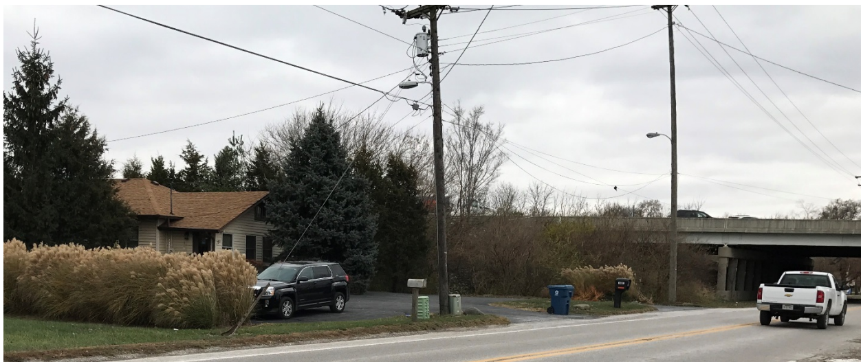
Figure 8-2: Views of 4401 Bluff Road with I-465 in Background
