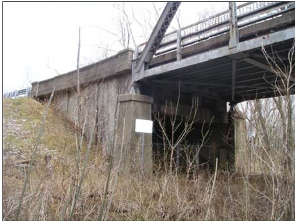
Figure 2. North side of bridge.
