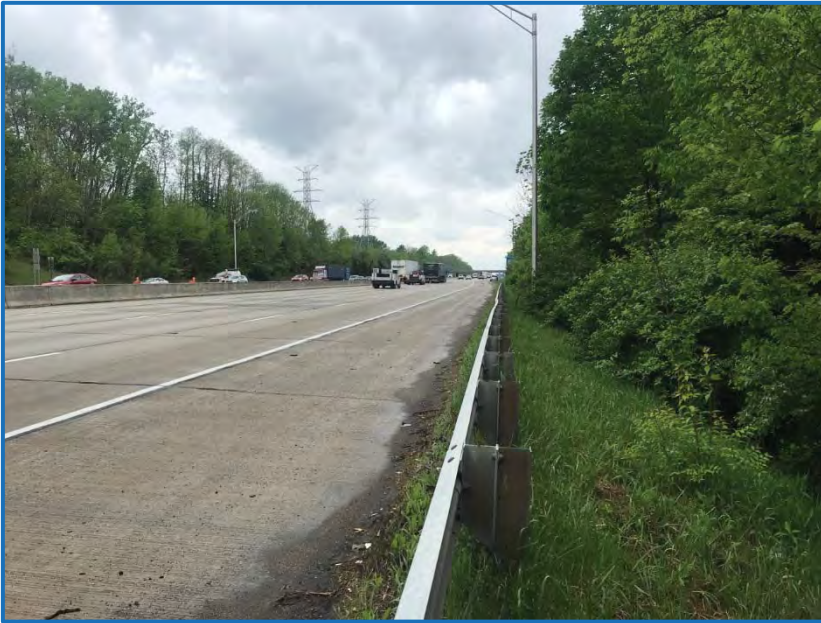
Photo 5 – View of roadside along westbound I-465 facing southwest (5-9-19).
