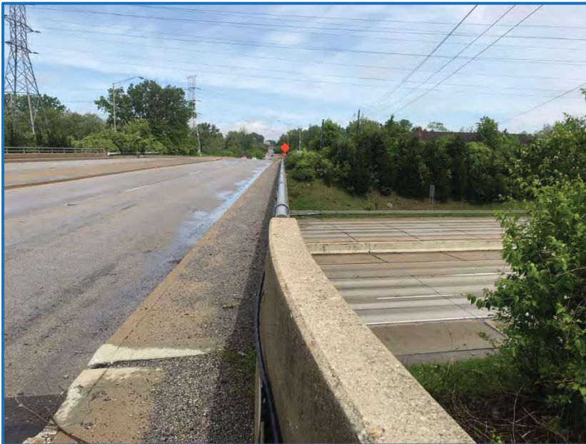
Photo 7 – View of Keystone Avenue bridge over I-465 facing north (5-22-19).
