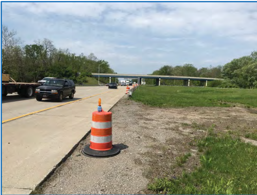
Photo 3 – View of roadside along eastbound I-465 facing west. Carson Avenue bridge is in the background (5-8-19).
