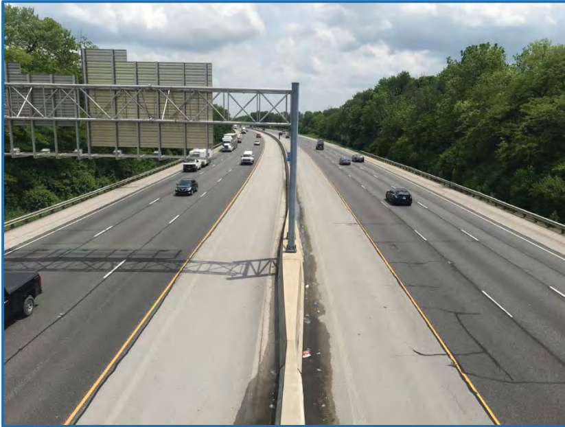
Photo 17 – View of I-465 from the Mooresville Road Bypass bridge facing southeast (5-24-19).
