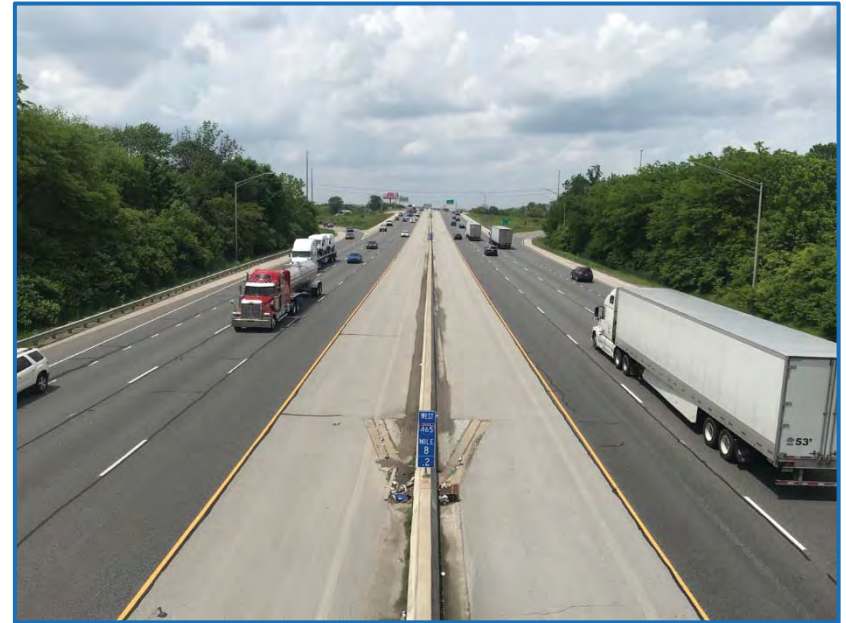
Photo 18 – View of I-465 from the Mooresville Road Bypass bridge facing northwest (5-24-19).
