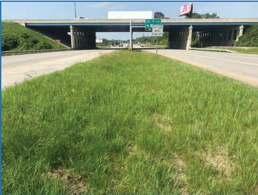
Photo 19 – View of Kentucky Avenue median north of the I-465 overpass facing south (5-28-19).
