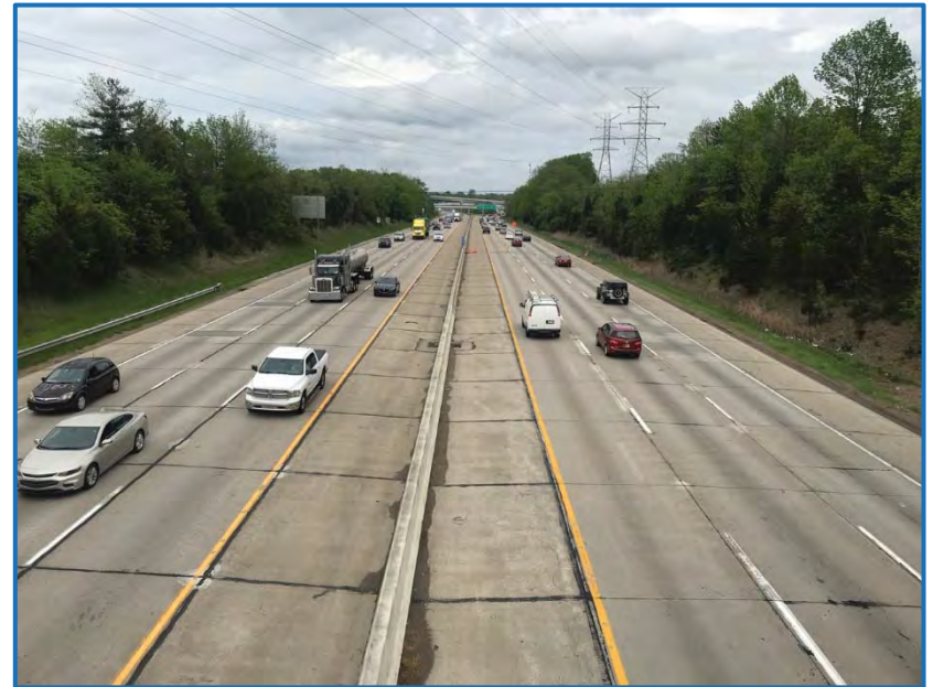
Photo 8 – View of I-465 from the Keystone Avenue bridge facing east (5-22-19).
