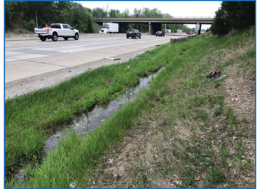
Photo 6 – View of roadside and Keystone Avenue bridge along westbound I-465 facing southwest (5-9-19).
