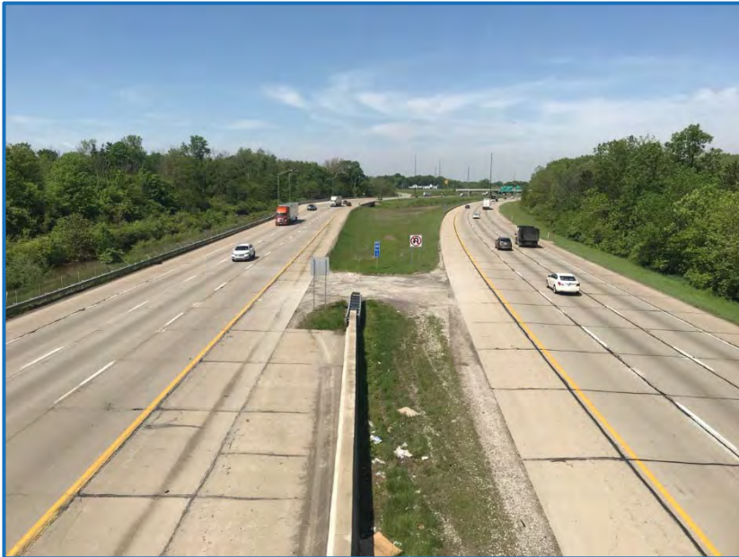
Photo 13 – View of I-465 from Madison Avenue bridge facing west (5-14-19).
