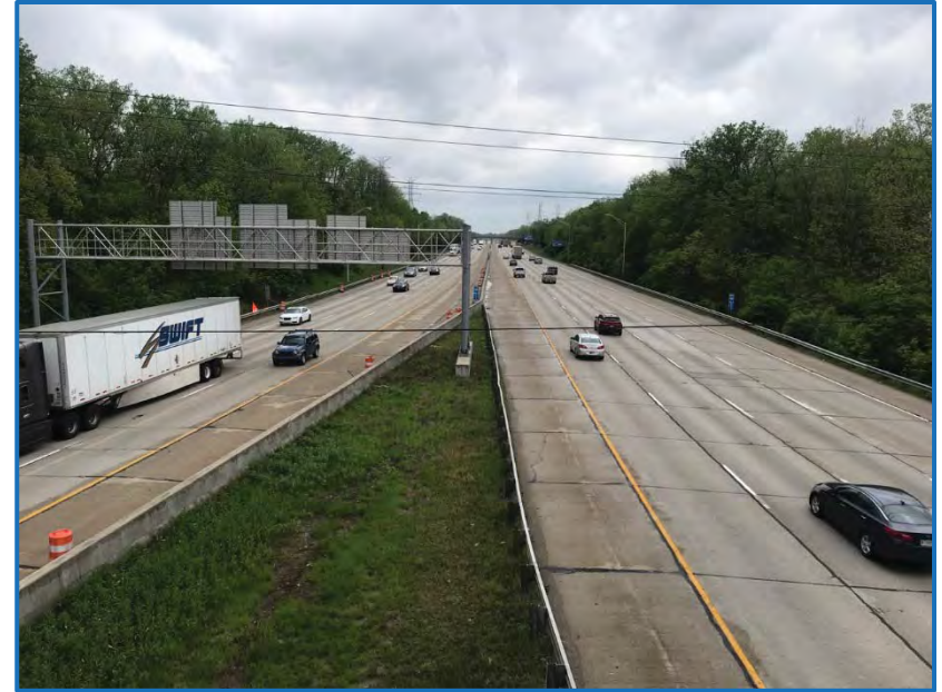
Photo 2 – View of I-465 from the Carson Avenue bridge facing west (5-9-19).
