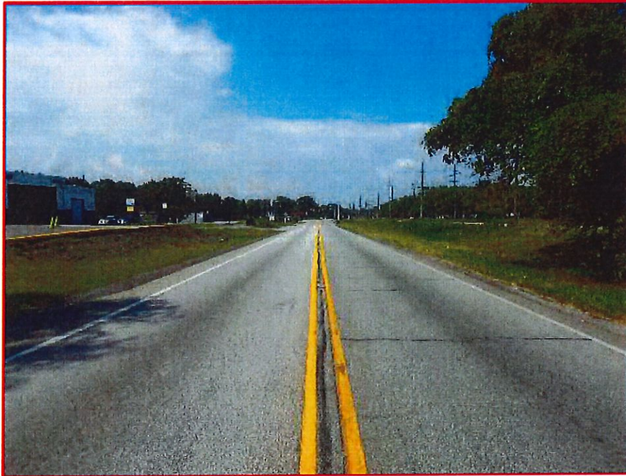
Photo 5: Looking southwest down US 12 from Clay Street.
