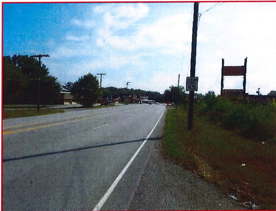
Photo 16. Looking east from southern edge of US 20.
