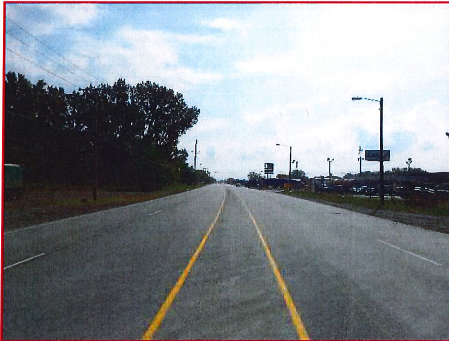
Photo 24. Looking east from eastern end of investigated area.
