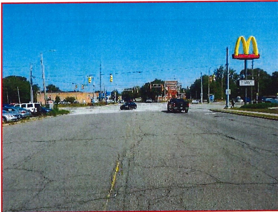
Photo 14. Looking north on Lake Street, north of US 20.
