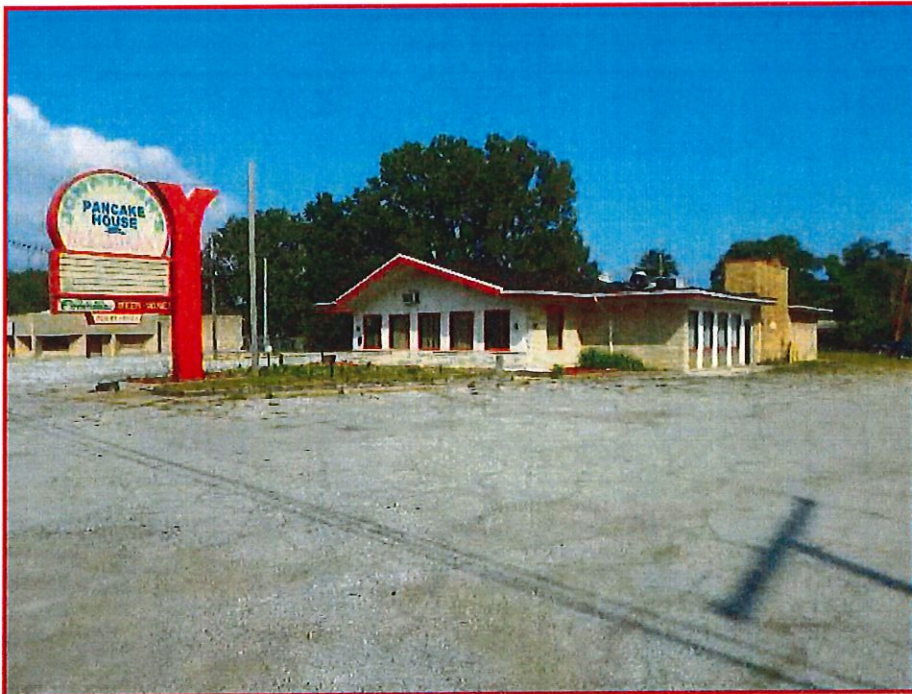
Photo 18. Looking northwest at Jonathan's Pancake House. Building to be removed.
