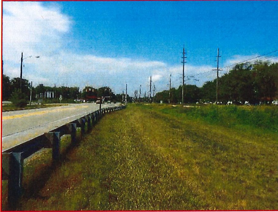
Photo 3. Looking southwest from northern edge of US 12.
