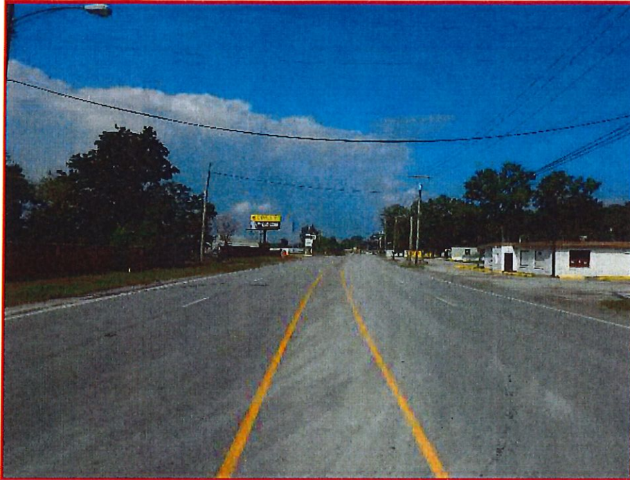
Photo 23. Looking west from eastern end of investigated area.
