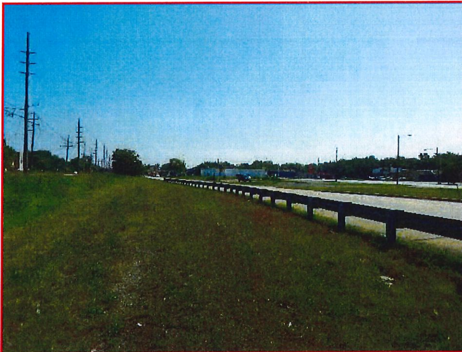
Photo 4. Looking northeast from northern edge of US 12.
