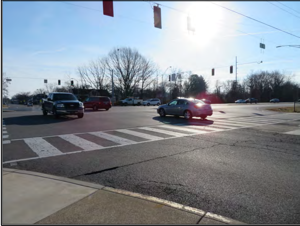
Figure B-2. Overview of project area at the intersection of US 41 and Washington Avenue, facing southeast.
