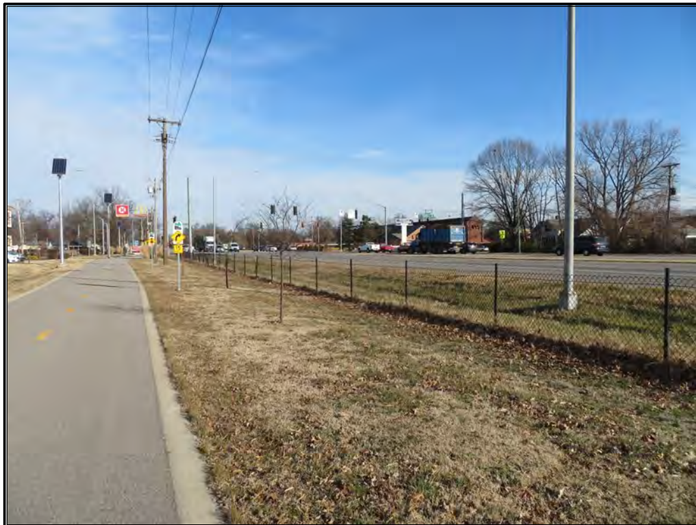
Figure 14. Overview of APE along US 41, facing northeast.
