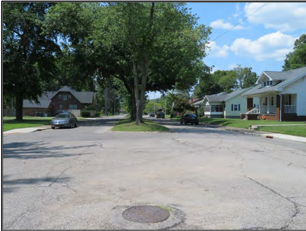
Figure 21. Overview of the Akin Park Historic District (IHSSI No. 163-196-430[01-213]) along Ravenswood Drive, facing southeast.
