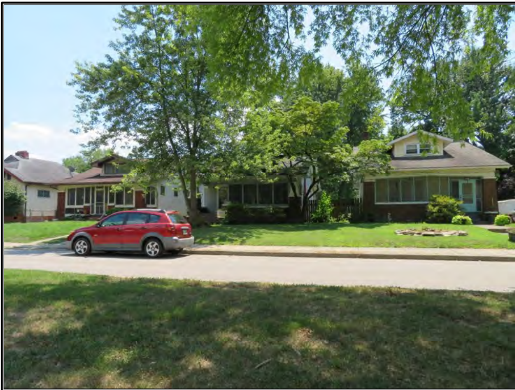
Figure 22. Overview of Akin Park Historic District (IHSSI No. 163-196-430[01-213]) along Taylor Avenue, facing southeast.
