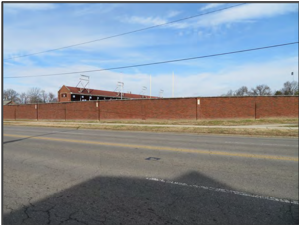
Figure 18. Exterior of Enlow Field (IHSSI No. 163-196-41044), part of the Lincolnshire Historic District (NR-0908) along Washington Avenue, facing northwest.
