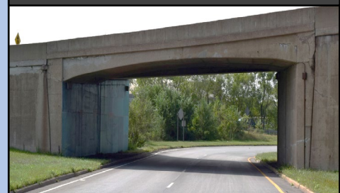
Figure 4: Ramp B over B bridge
