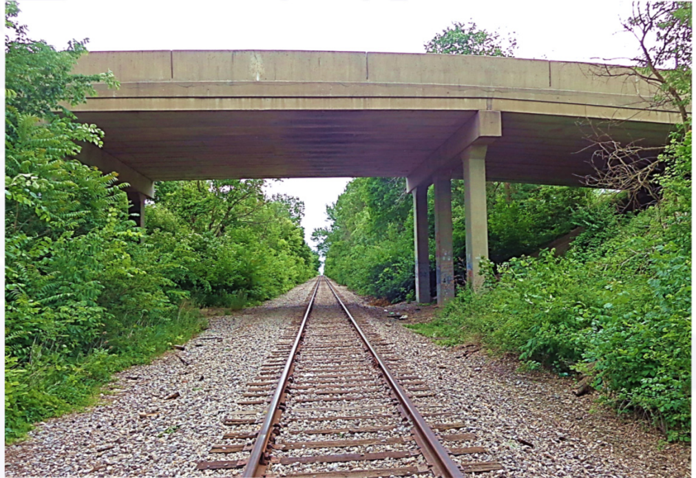
Looking east at the Main Street bridge
