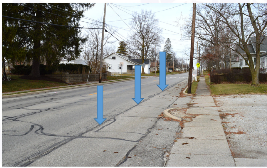
Looking north along SR 22 (Main Street)
