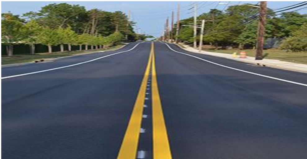
Figure 1. New pavement markings.
